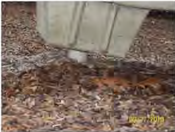
A lack of wood fiber play surfacing is evident at the base of this slide. Wood fiber has been replenished as budget allows, but all playgrounds require more for adequate safety and accessibility.
