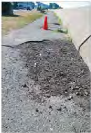
Sinkholes and deterioration of walkway pose safety hazards at Joppa Park; benches need replacement; lawn needs replacement.
