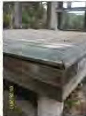
Wooden sandbox structure needs repair with decking lifting up and a wooden ramp falling off.
