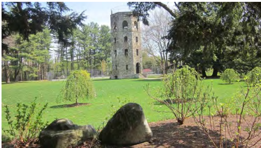
Stone tower at Atkinson Common
