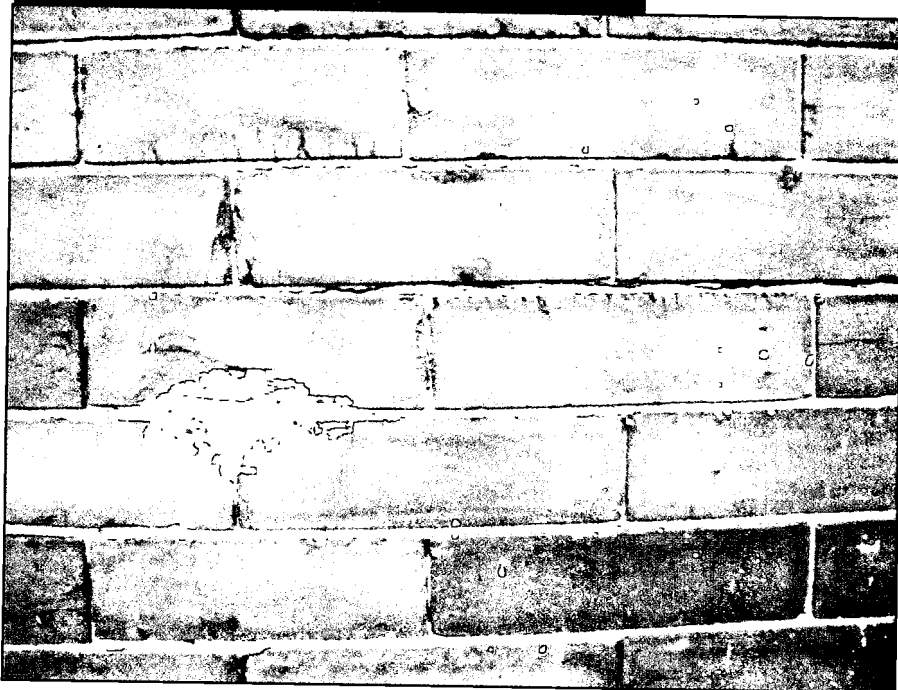
Photo J: North Façade Running Bond Pattern
