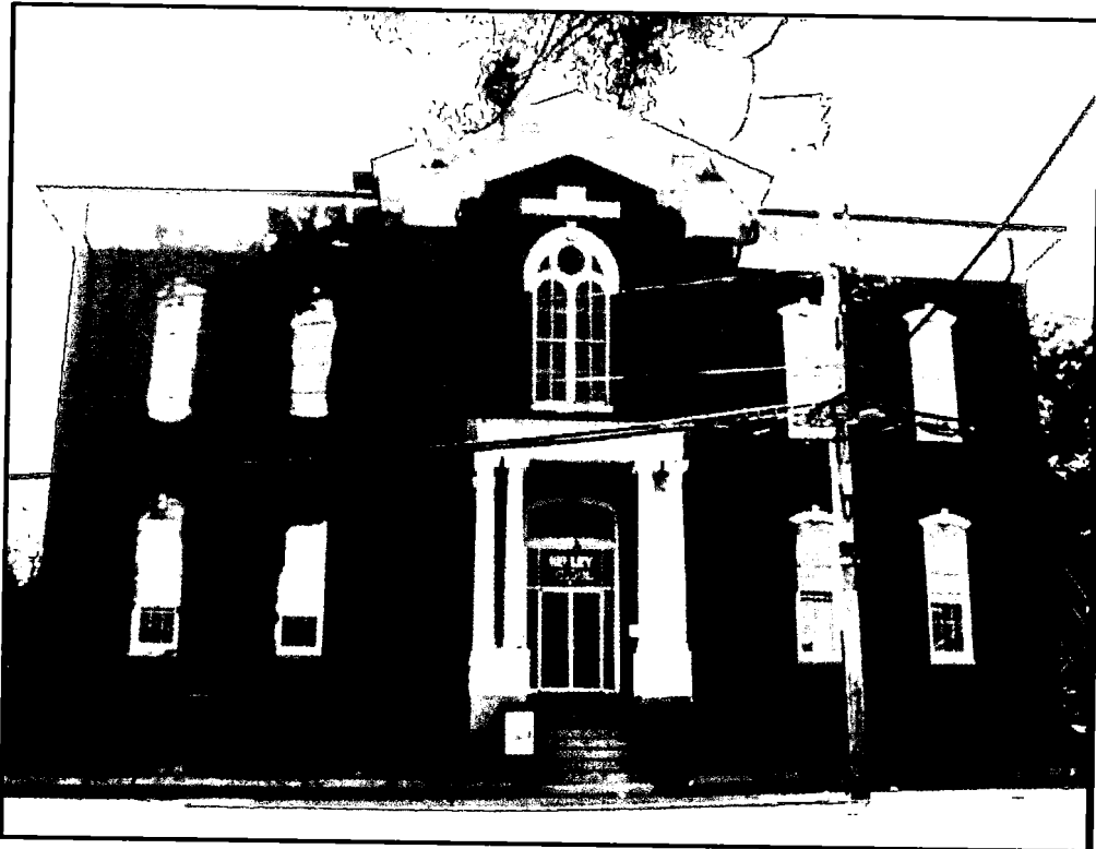
Photo K: North Façade – High Street
