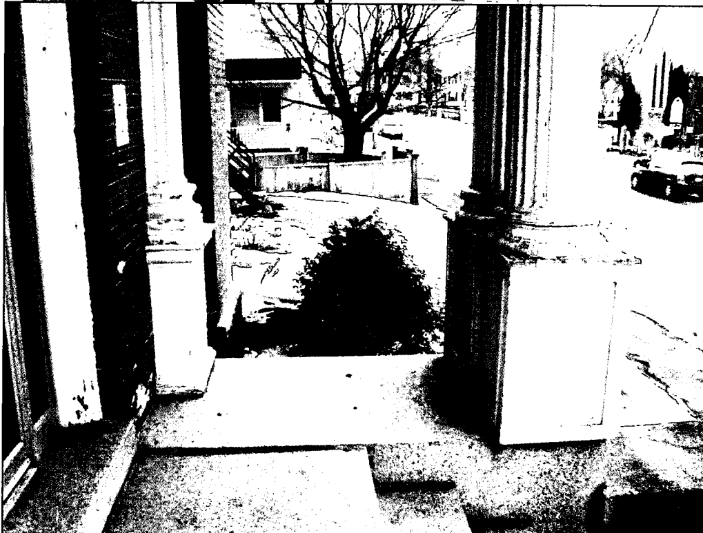
Photo F: Detail – Base of Portico Columns
