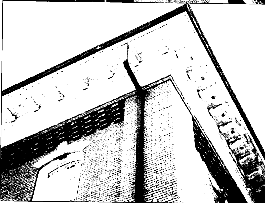
Photo B: South East Façade Cornice Detail
