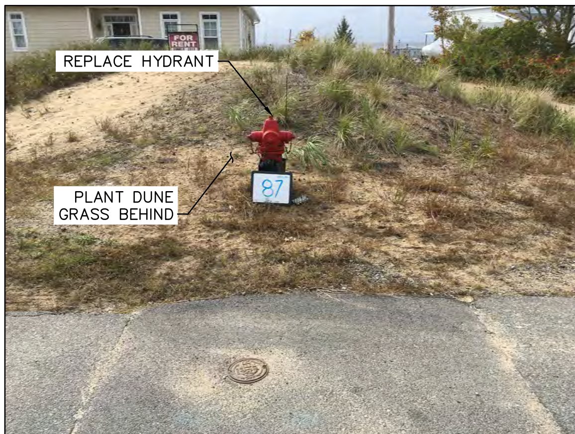
HYD-87 BASIN STREET @ HARBOR STREET
