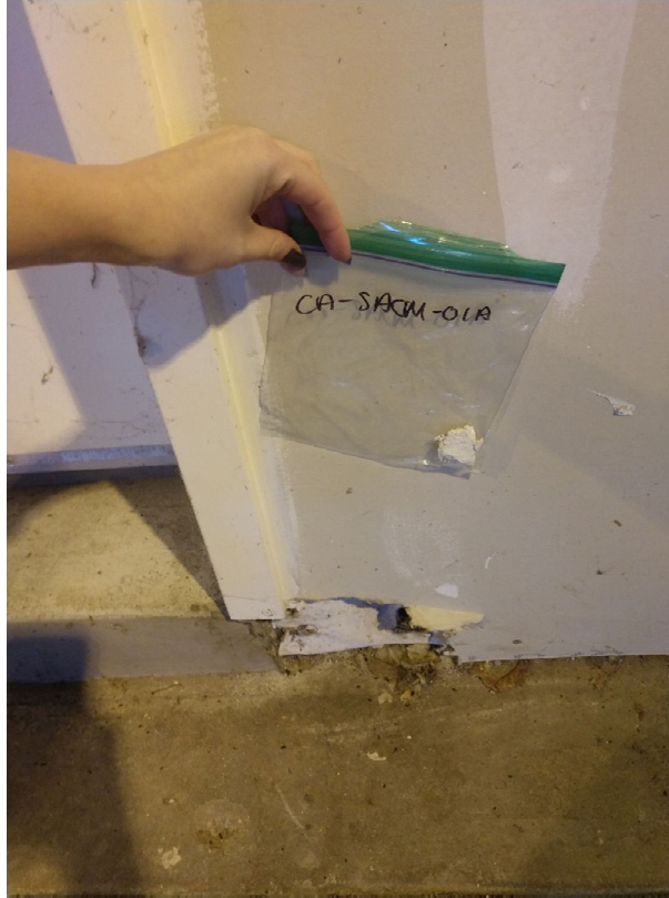
1. Material CA-SACM-01, light gray sheetrock found throughout the building
