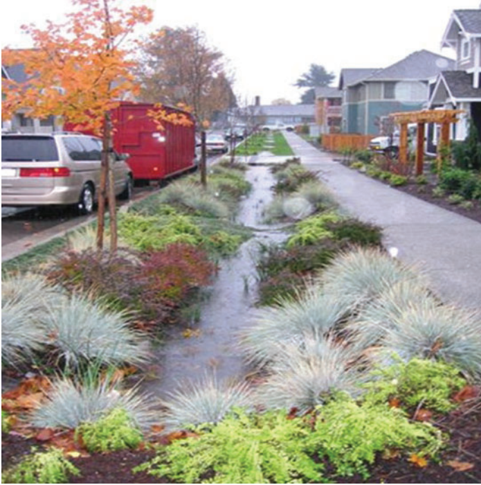
Figure 5 Surface raingarden channel for clean water /stormwater and pond outlet flow during rainfall in Malmö Sweden.
