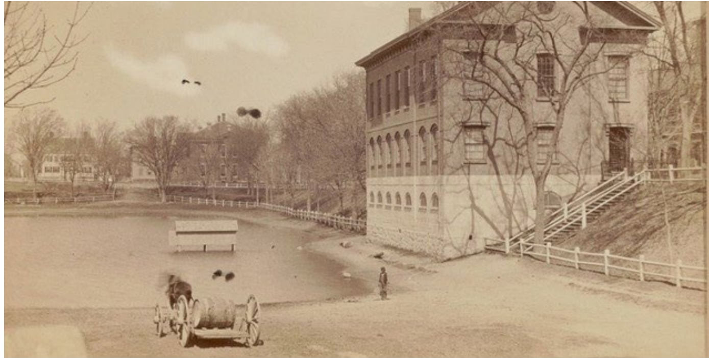
Fire shed in middle of pond
