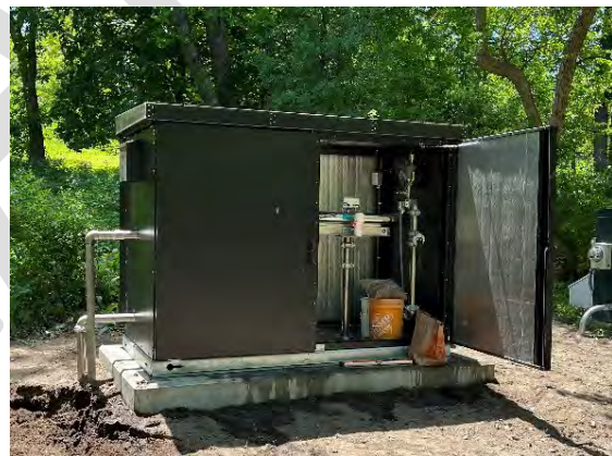
Figure 19: Prefabricated Pump Station Enclosure (During Construction)
