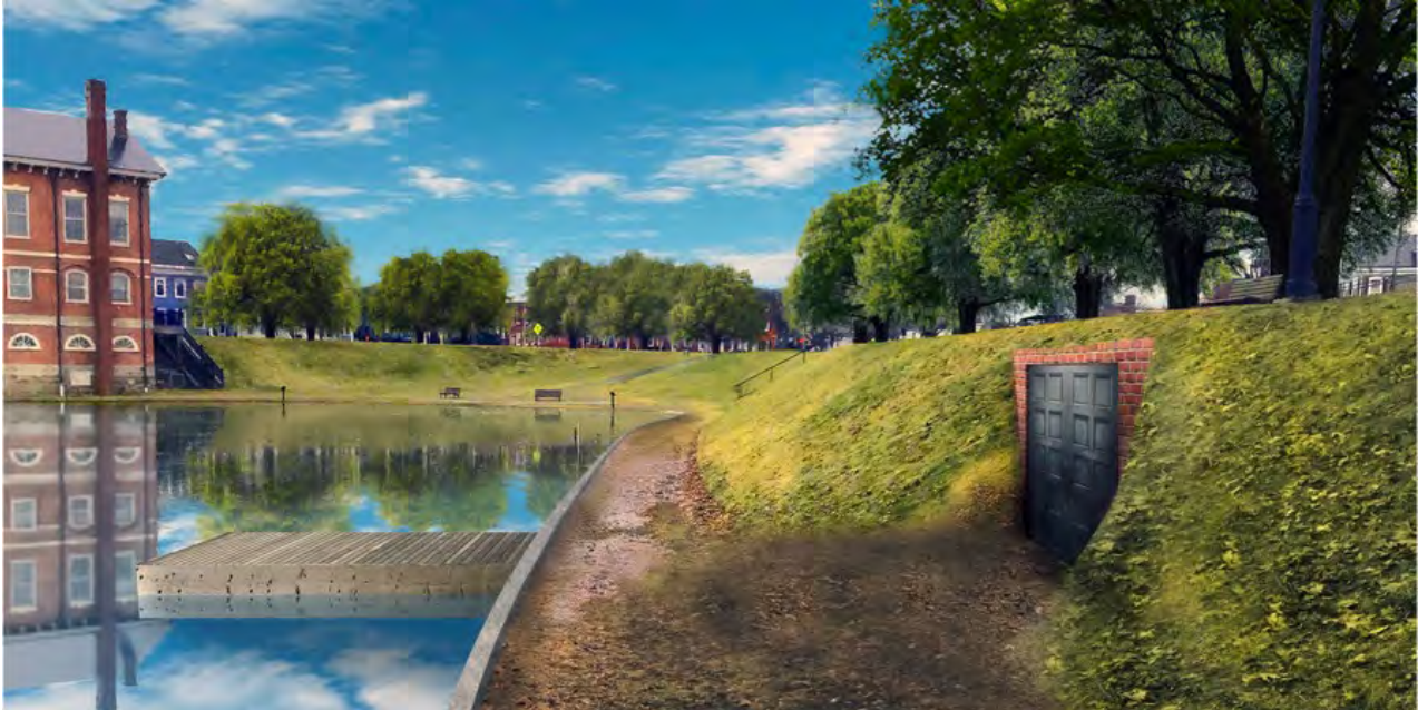
Figure 9: Frog Pond Underground Pump Station
