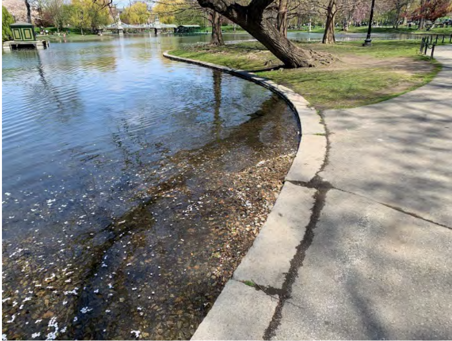
Figure 8: Granite Curbing Circumscribing Boston Public Garden Lagoon (Shallower Curb Height and Pond Depth than Proposed for Newburyport Frog Pond)
