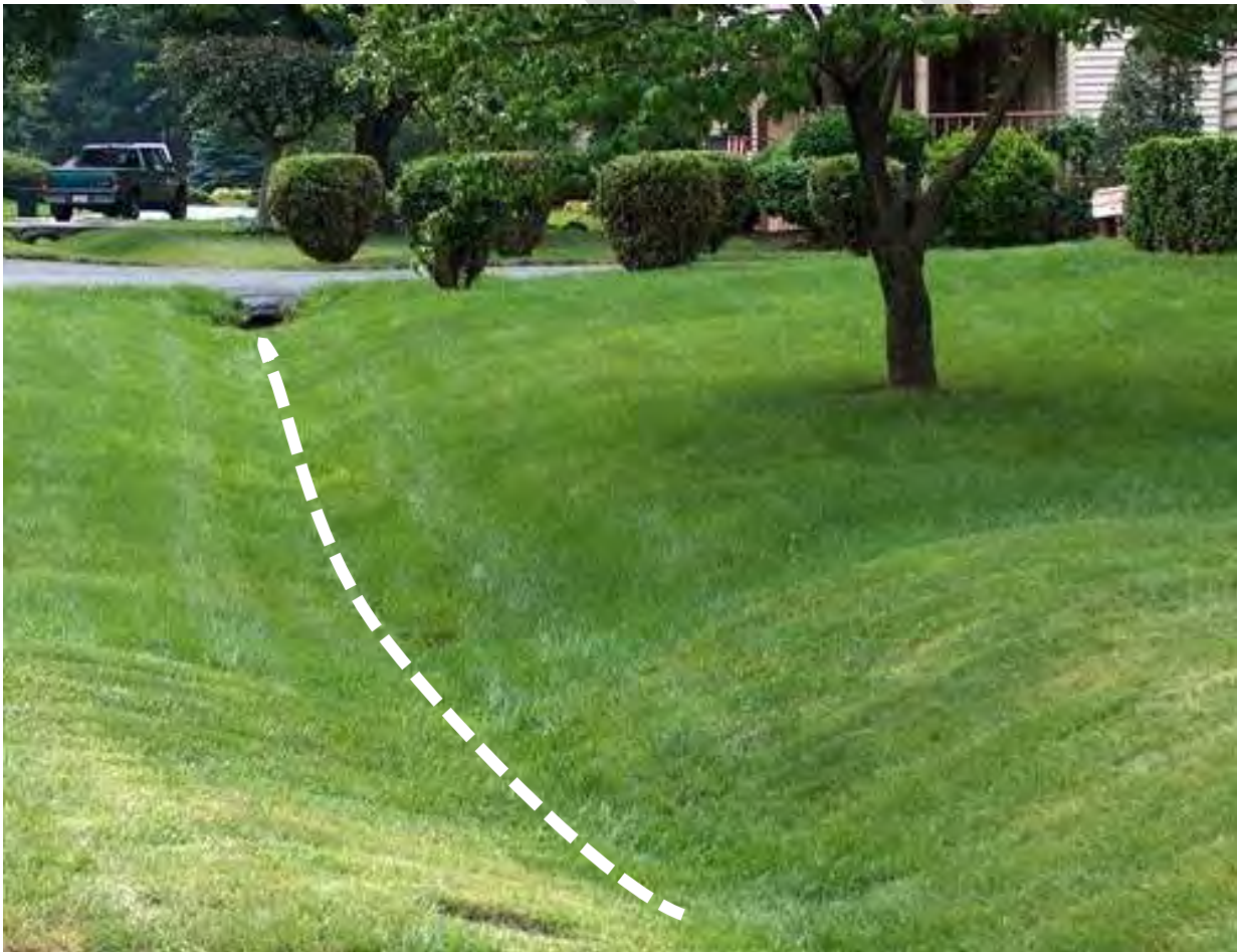
Figure 20: Typical Grass Swale Collecting Runoff from Each Side (Dashed Line is Bottom of Swale to Infiltration)
