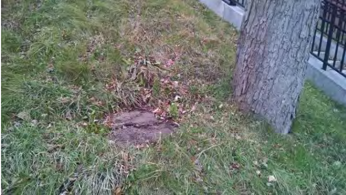
Figure 3: Valve Location next to Courthouse Steps
