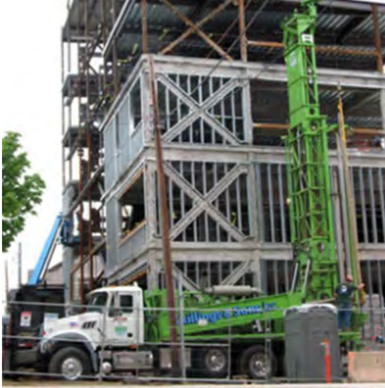
Figure 14: Typical Drilling Rig (Courtesy of Skilling & Sons Drilling, New Hampshire)
