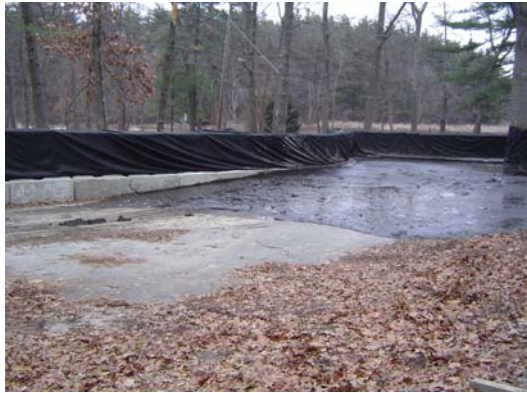
Photo 2. Sediment immediately after dredging.
