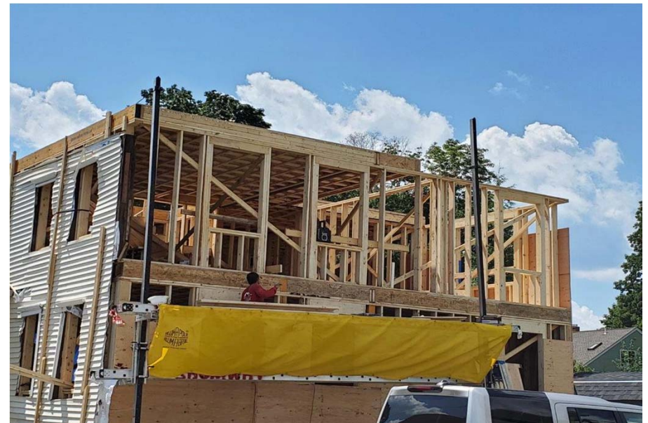
12-14 Harrison Street (original framing and sheathing is also protected)
