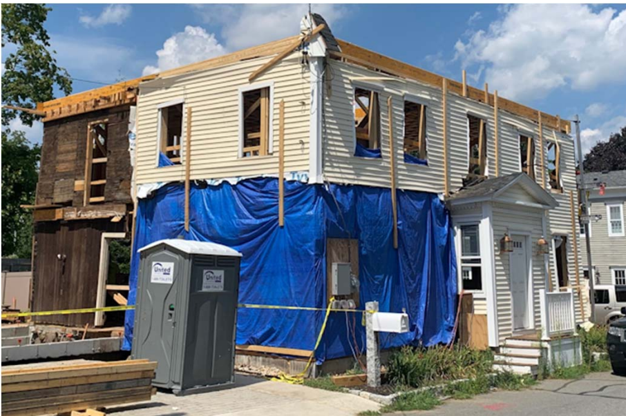
12-14 Harrison Street (original framing and sheathing is also protected)
