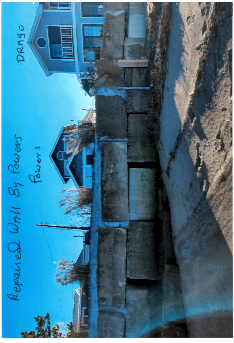
Existing Wall City owned in Need of Repair Undermining
