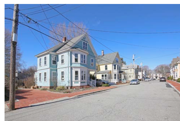
STREET VIEW: NORTHEAST CORNER
