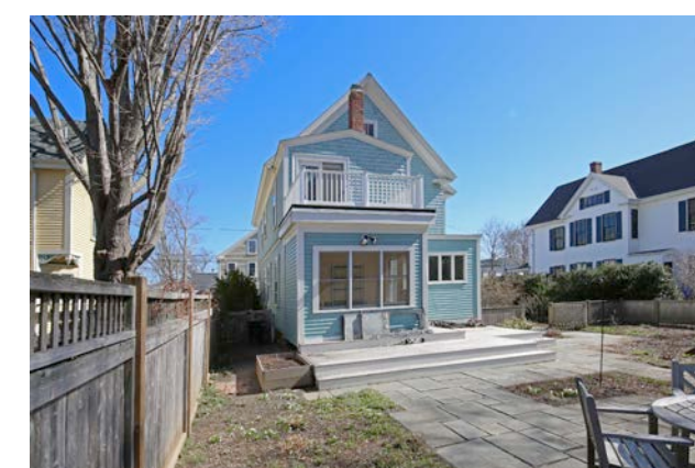
REAR VIEW: SOUTHWEST CORNER
