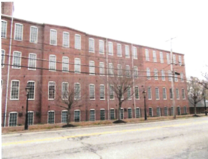
West elevation, view southeast
