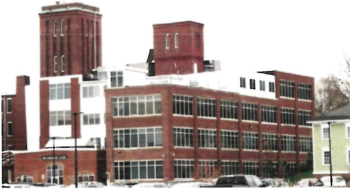
East elevation on left, north elevation on right, view southwest
