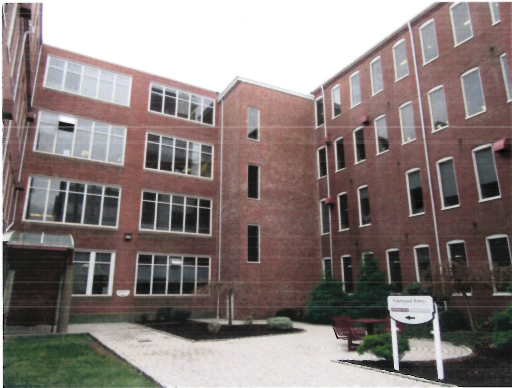
12. View south of courtyard
