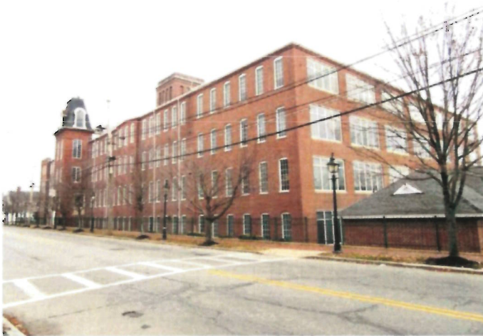
View east, west elevation on left, south elevation on right
