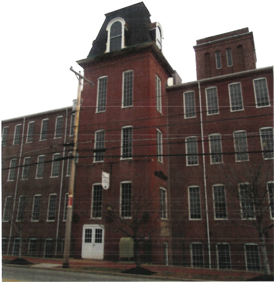
3. Façade, detail of stairtower
