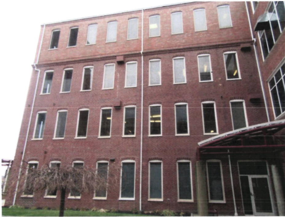
13. View east of courtyard
