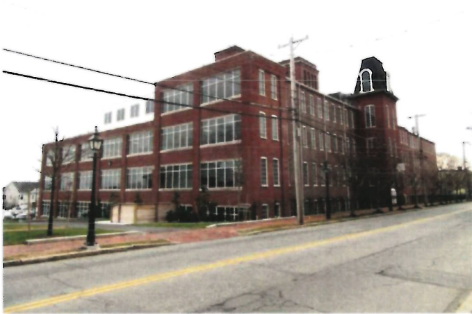
North elevation on left, west elevation on right, view southeast
