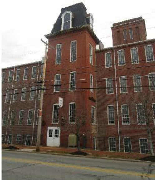
11. West elevation of 1866 building, view east at center
