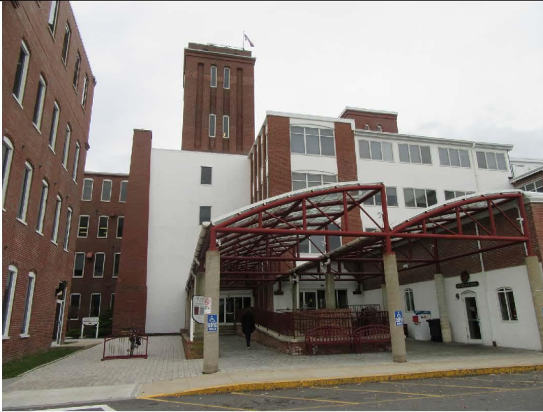
24. East elevation of EFIS addition, detail at entrance, view west
