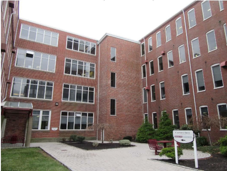
25. Courtyard, west elevation of 1947 addition, east elevation of 1866 building on right, view southwest
