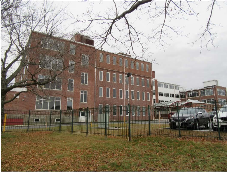
26. East elevation of 1947 addition on left, east elevation of 1866 building on right, view northwest
