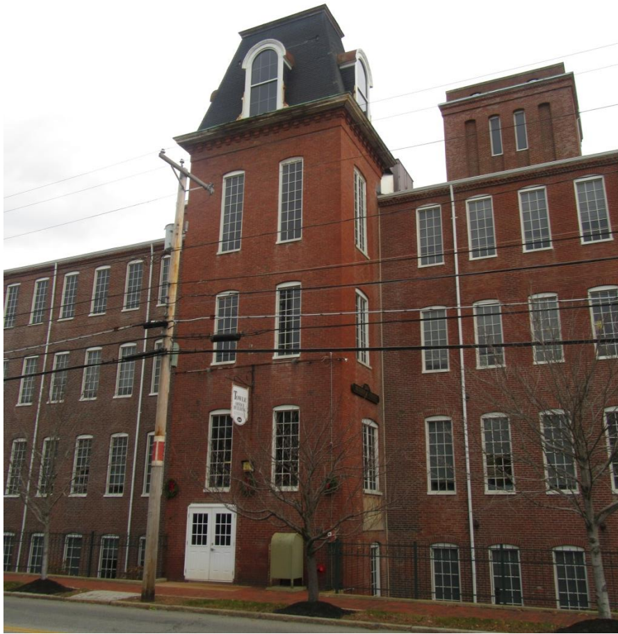
3. Façade, detail of stairtower
