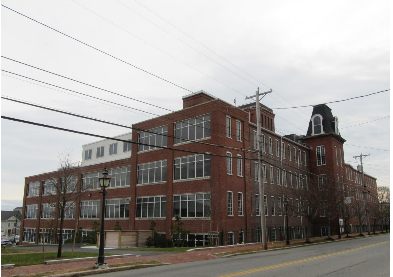
2. West elevation (façade), left and north elevation, right.
