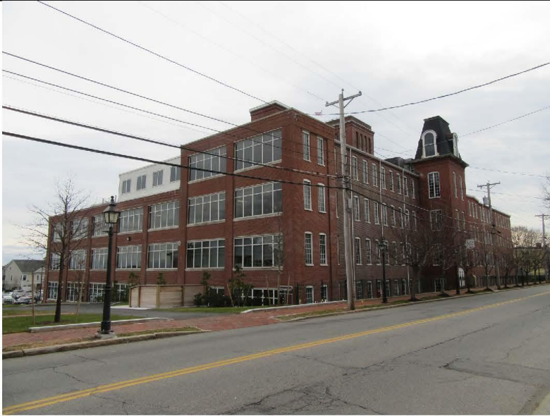
18. North elevation of c. 1926 addition on left, west elevation of 1866 building and 1926 addition on right, view southeast
