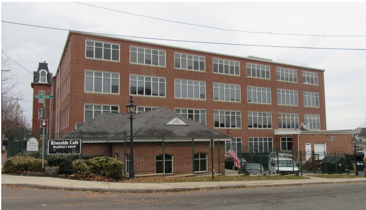
4. South elevation of Towle Building. South elevation of Maintenance Building (foreground).
