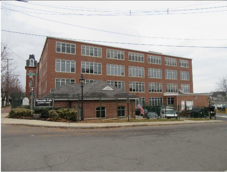
28. South elevation of 1947 addition, view north
