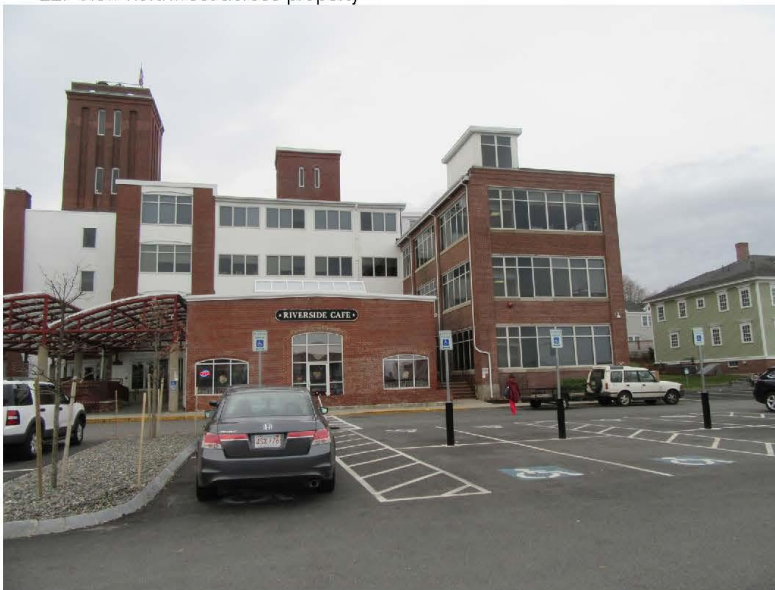
23. North end of east elevation of complex, view west
