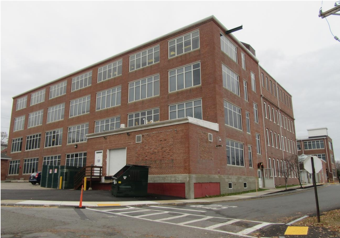
5. South elevation, left and east elevation, right
