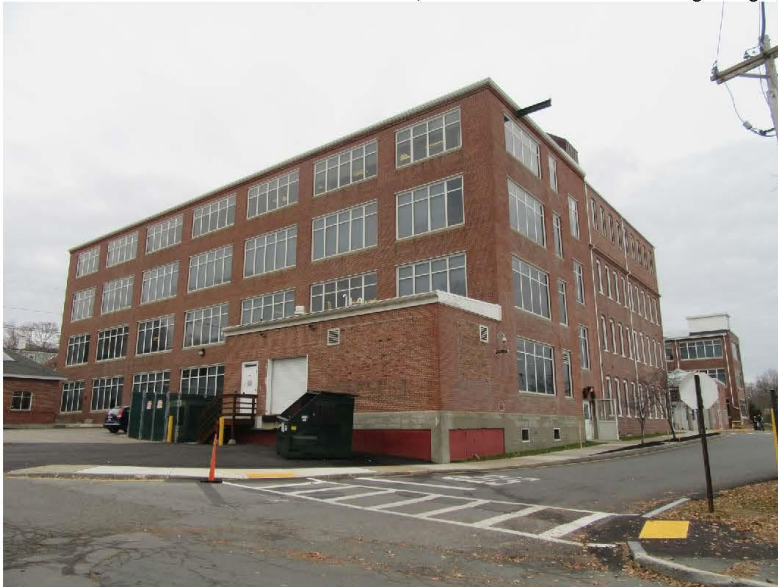
27. South elevation of 1947 addition on left, east elevation of 1947 addition and 1866 building on right, view northwest
