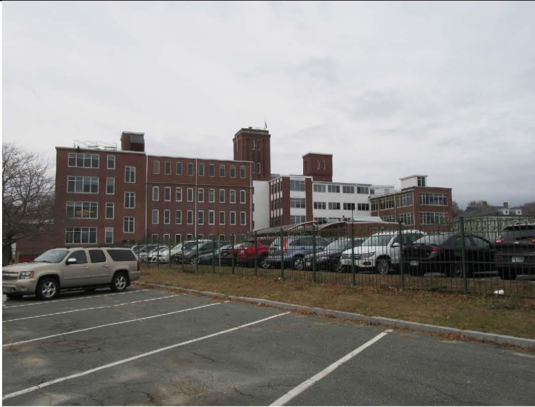
22. View northwest across property
