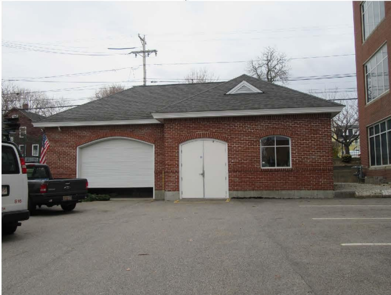
29. East elevation of maintenance building, view west
