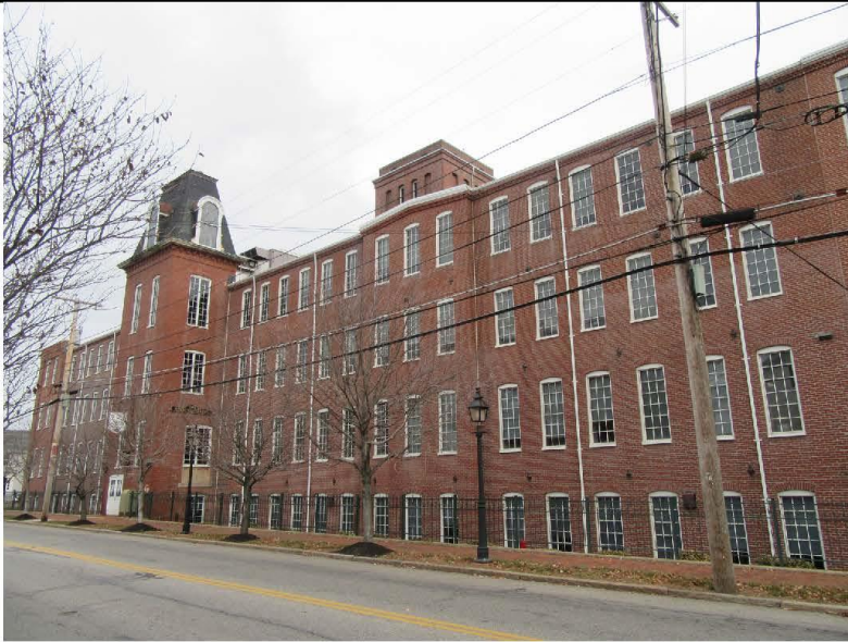
16. West elevation of 1866 building, view northeast
