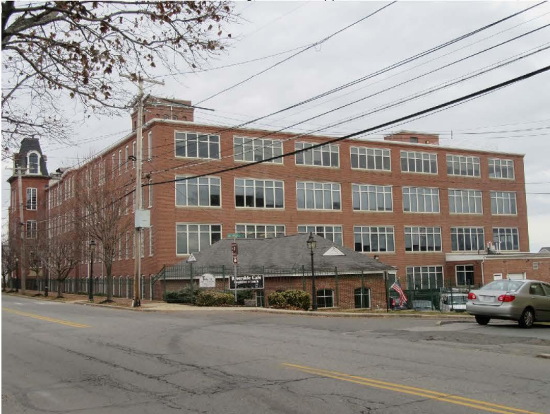
13. West elevation of 1866 building on left, south elevation of 1947 building on right, view northeast
