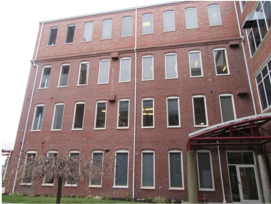
13. View east of courtyard
