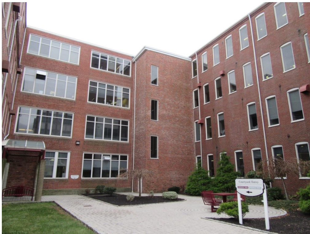
12. View south of courtyard
