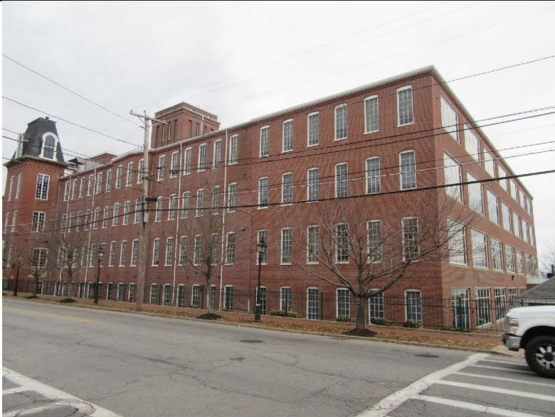
14. West elevation of 1866 and 1947 buildings on left, south elevation of 1947 building on right, view northeast
