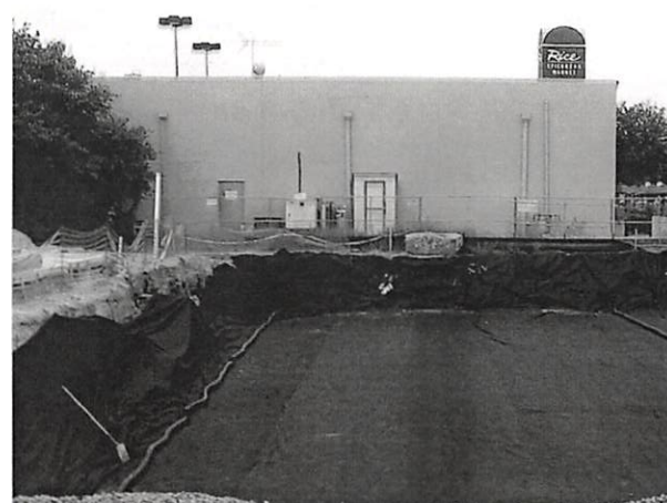
Place non-woven geotextile over prepared soils and up excavation walls.
