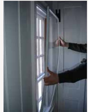
Interior storm panel.
