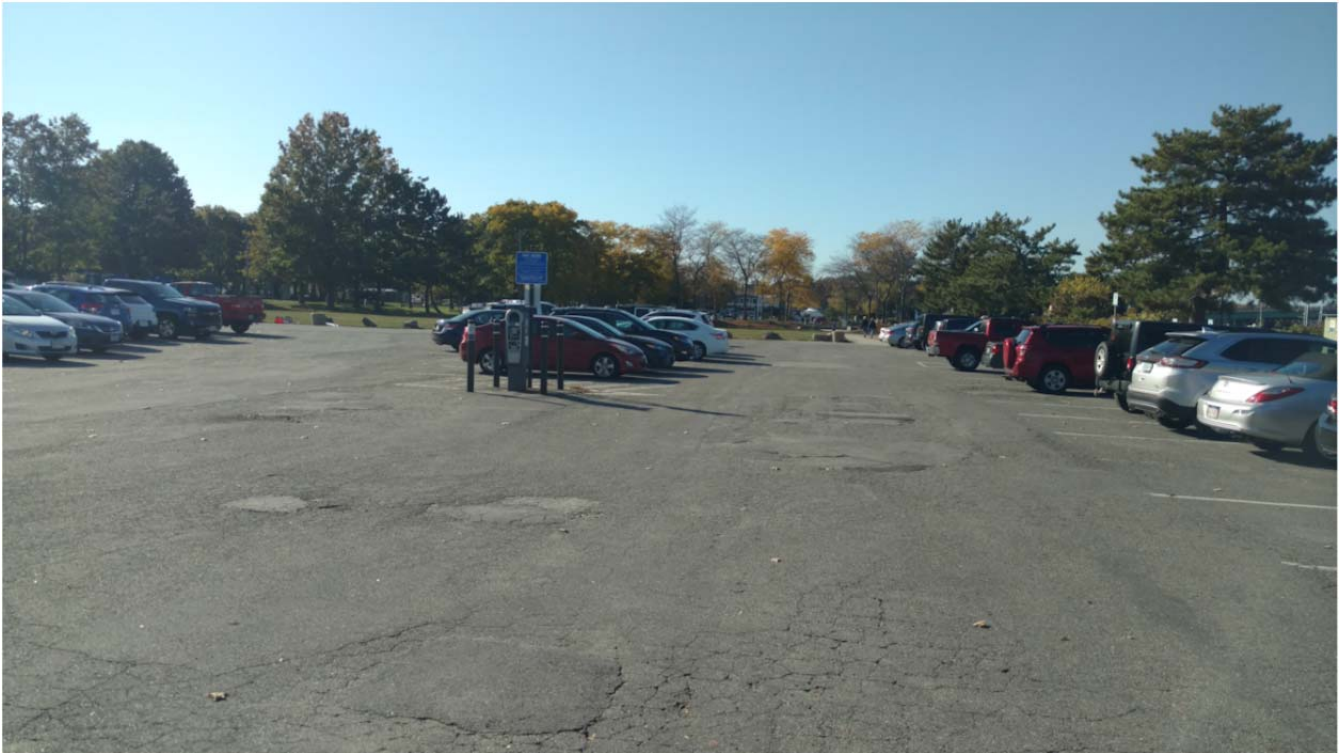
View West across East Lot/Parking
