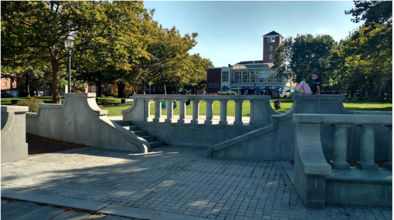
Granite Walls, Steps & Ramps, View from Central Embayment, Market Landing Park
