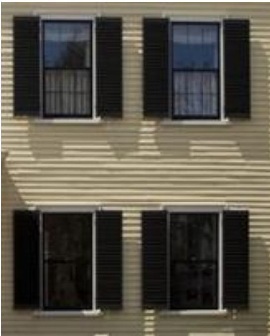
Figure 6 – Example of Federal-Style Shutters
