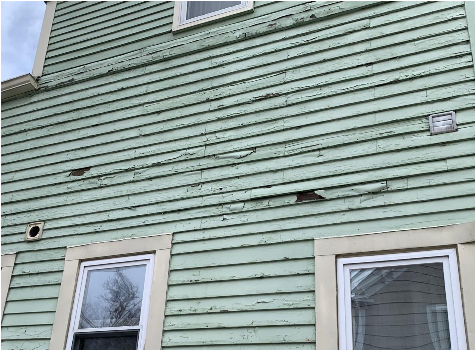
Figure 8B – Clapboard Repair
