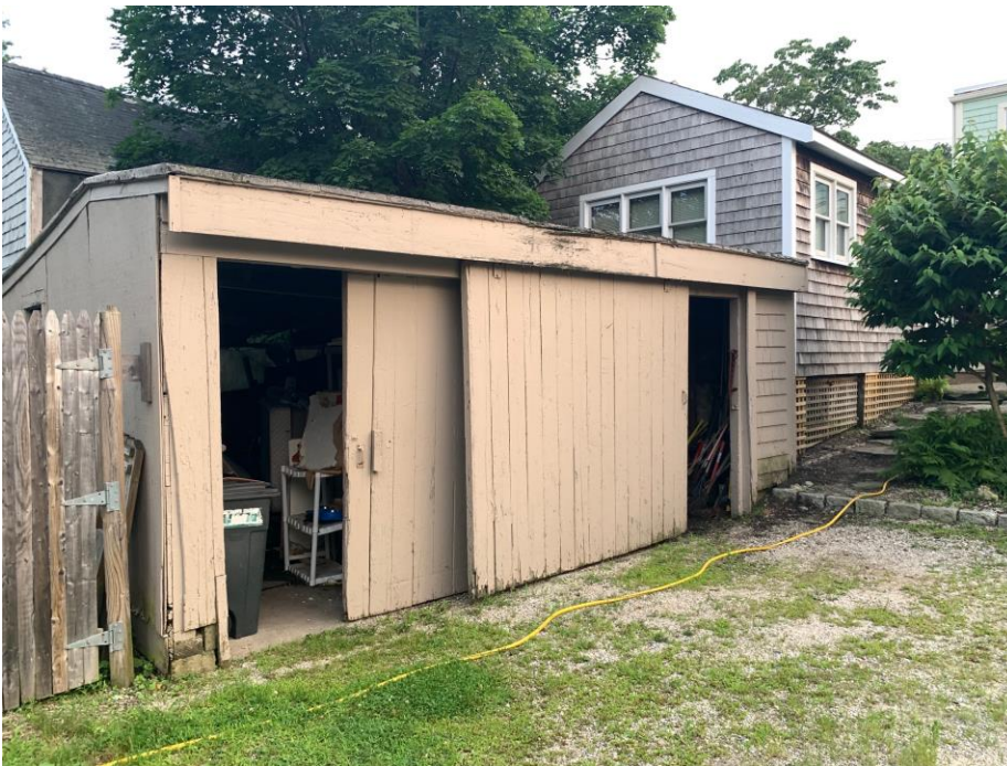
Figure 10 – Rear Shed to be Removed
