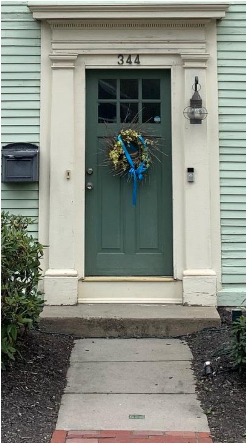
Figure 5 – Walkway Preservation and Step Replacement
