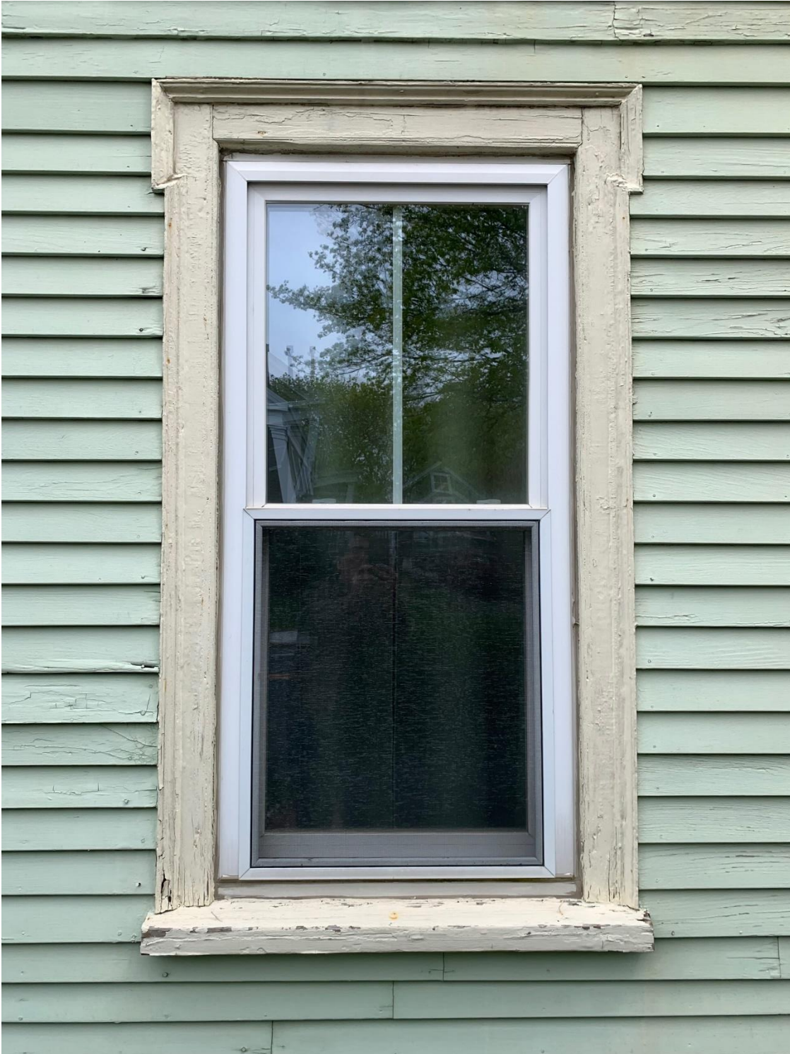
Figure 2 – Existing Window Casing on the Merrimac Street Facade
