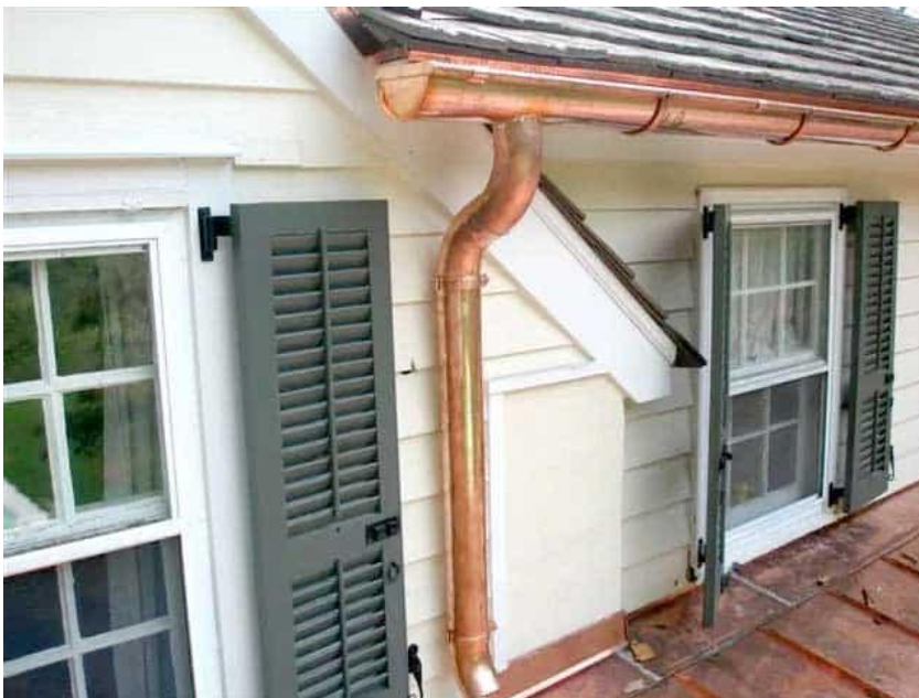
Figure 7 – Examples of Gutters and Downspouts
