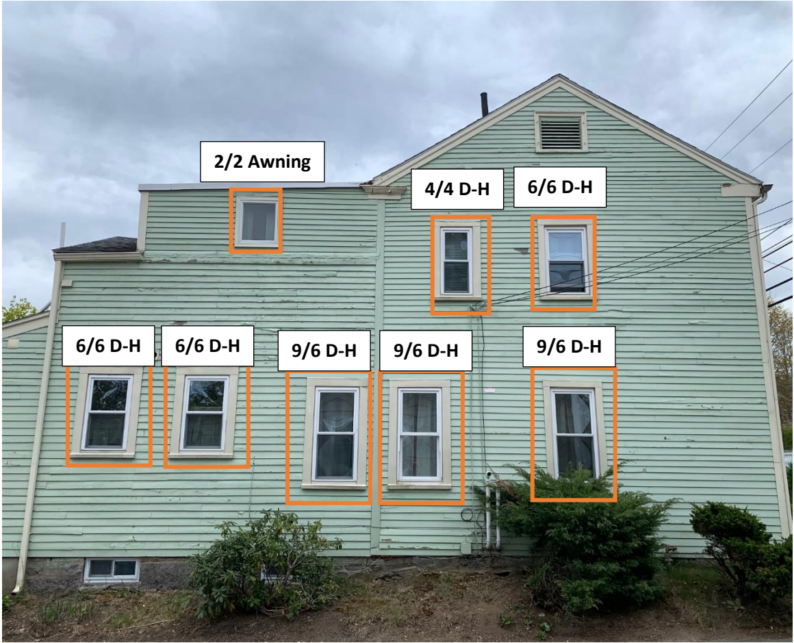
Figure 1B - Window Replacement on the Union Place Facade
