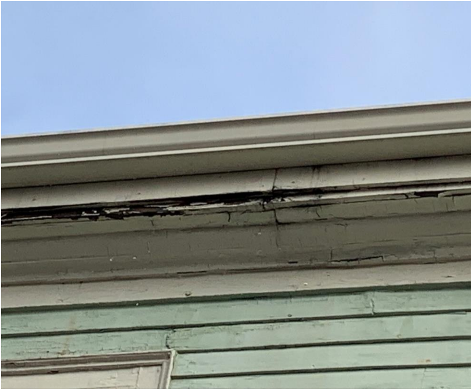
Figure 8A – Soffit and Trim Repair
