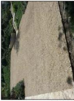
Chip Seal Driveway
