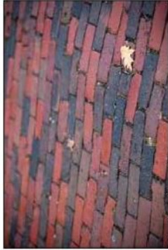
Clay Brick Sidewalk
