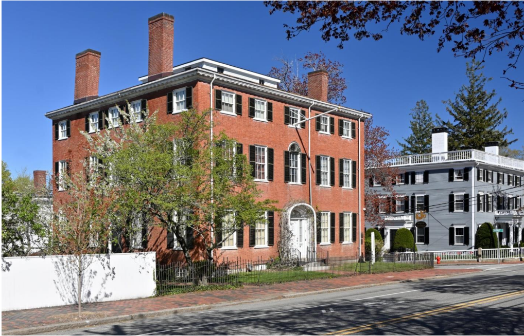
c. Photo 3: North and West Elevations Cushing House 2021
