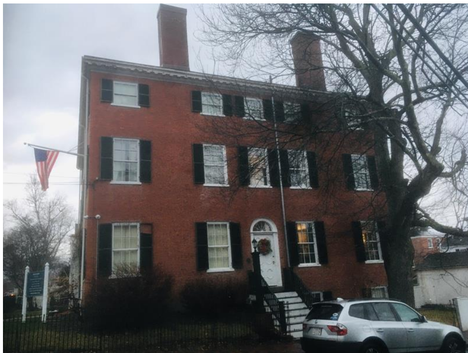
f. Photo 6: East Elevation, Cushing House, January 2022
