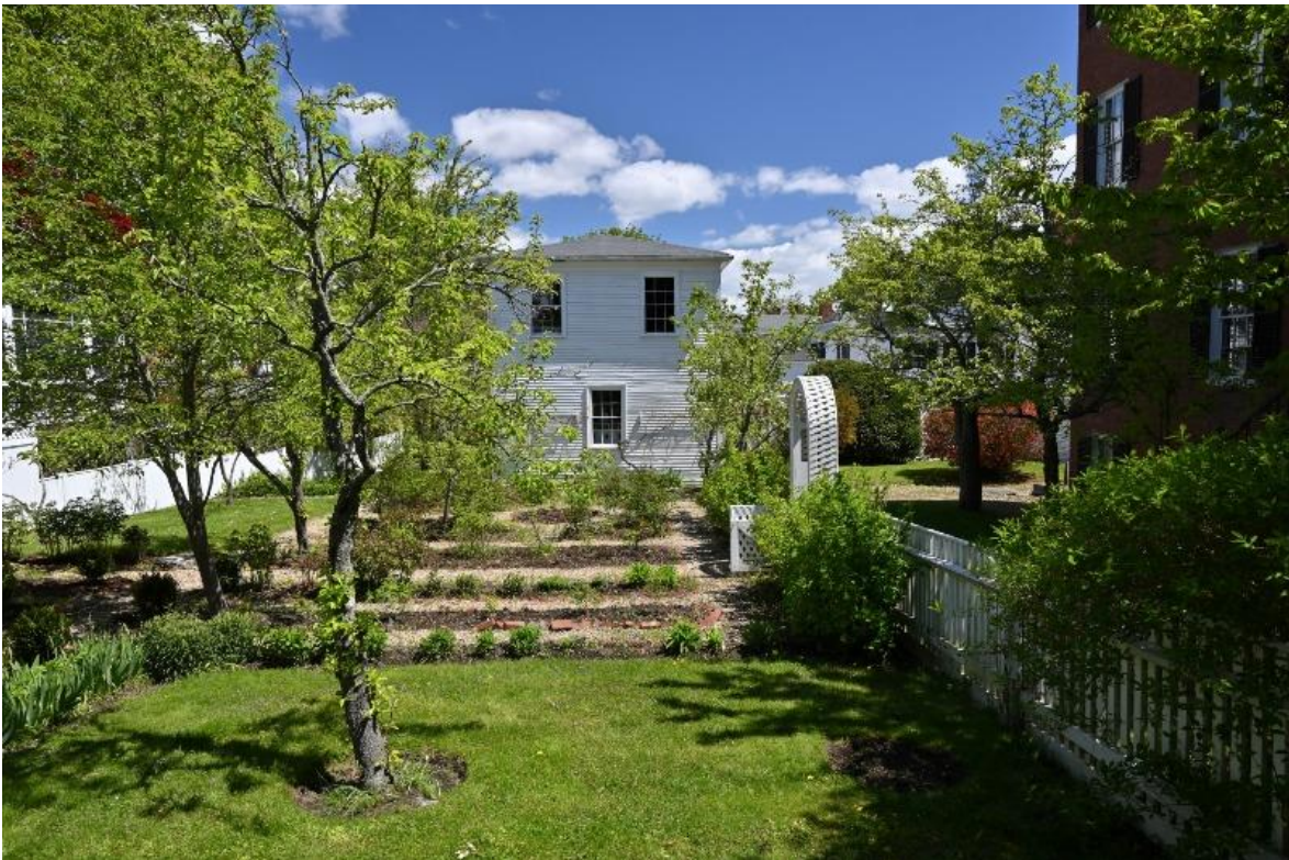
k. Photo 11: North elevation Carriage Barn, Cushing House, May 2021
