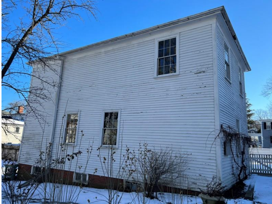
1. Photo 12: Rear Elevation, Carriage Barn, Cushing House, January 2022
