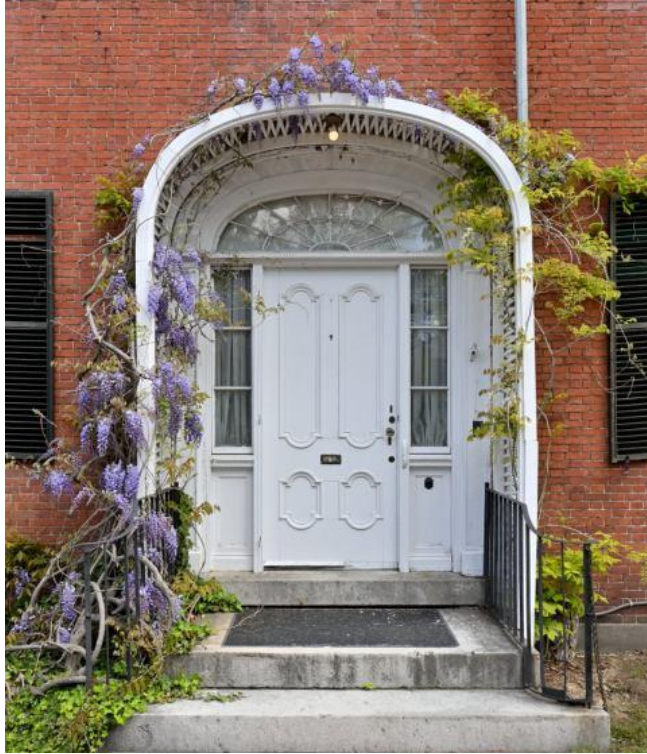
g. Photo: 7 Main Entry Detail - North Elevation, Cushing House, June 2021
