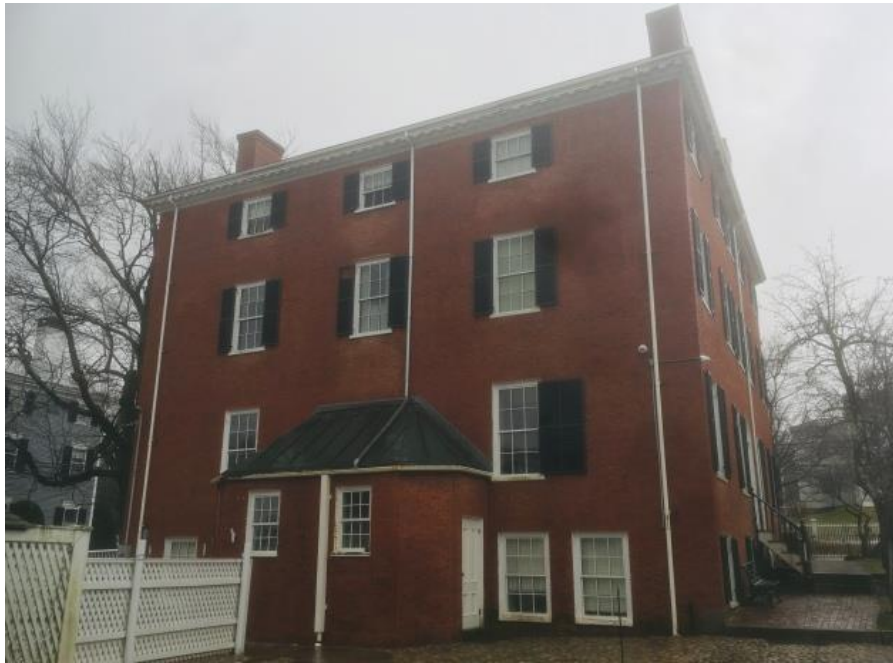
e. Photo 5: South Elevation, Cushing House, January 2022
