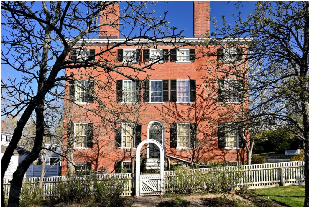
d. Photo 4: West Elevation, Cushing House, May 2021
