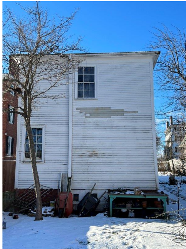
m. Photo 13: South Elevation Carriage Barn, Cushing House, January 2022
