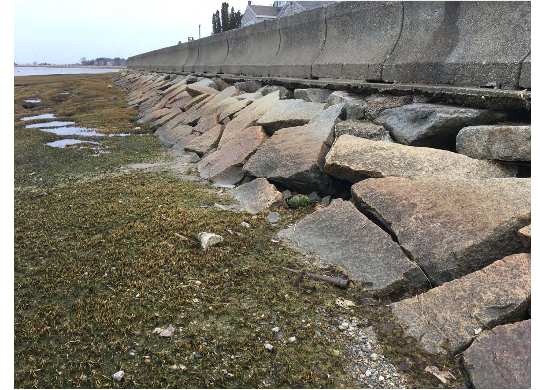
View along seawall
