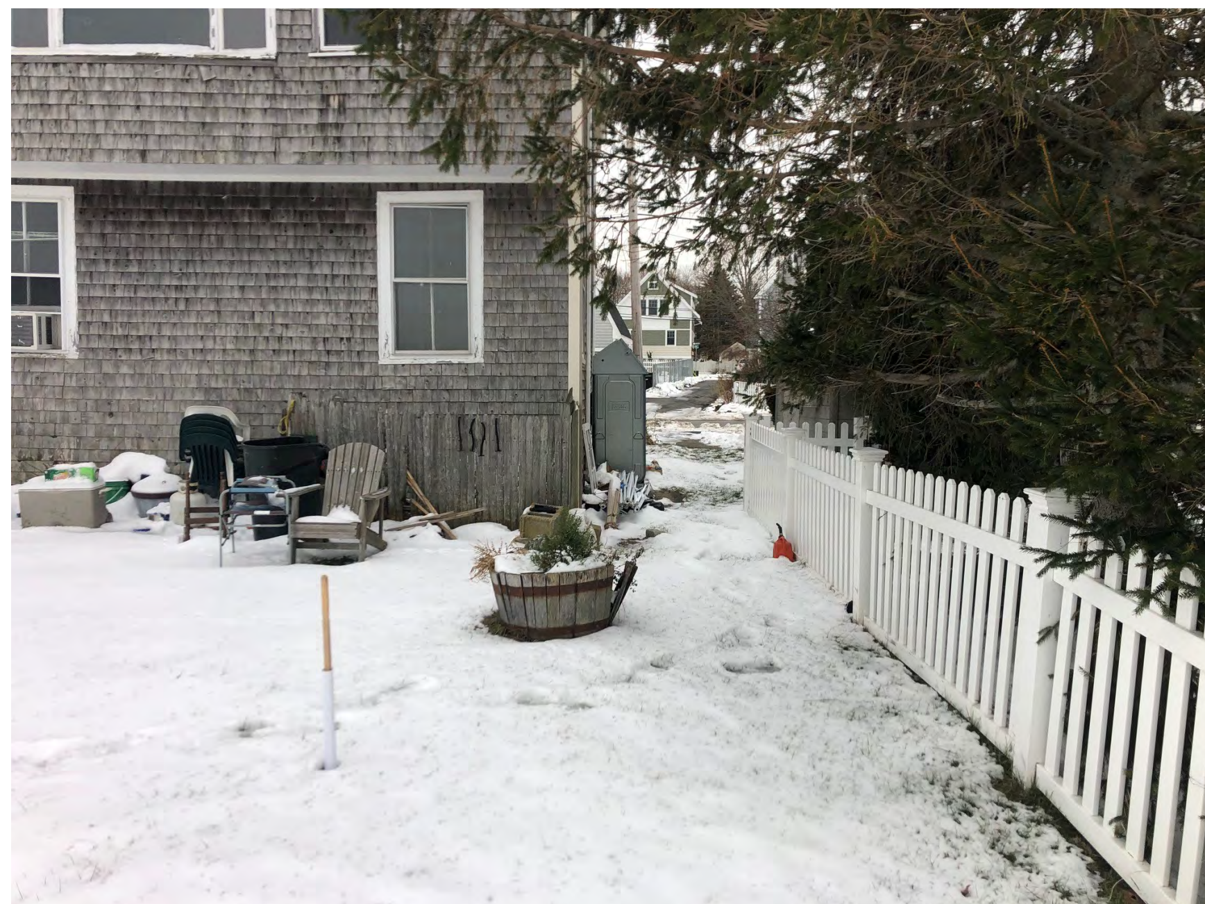
Water side of existing building View along wall
