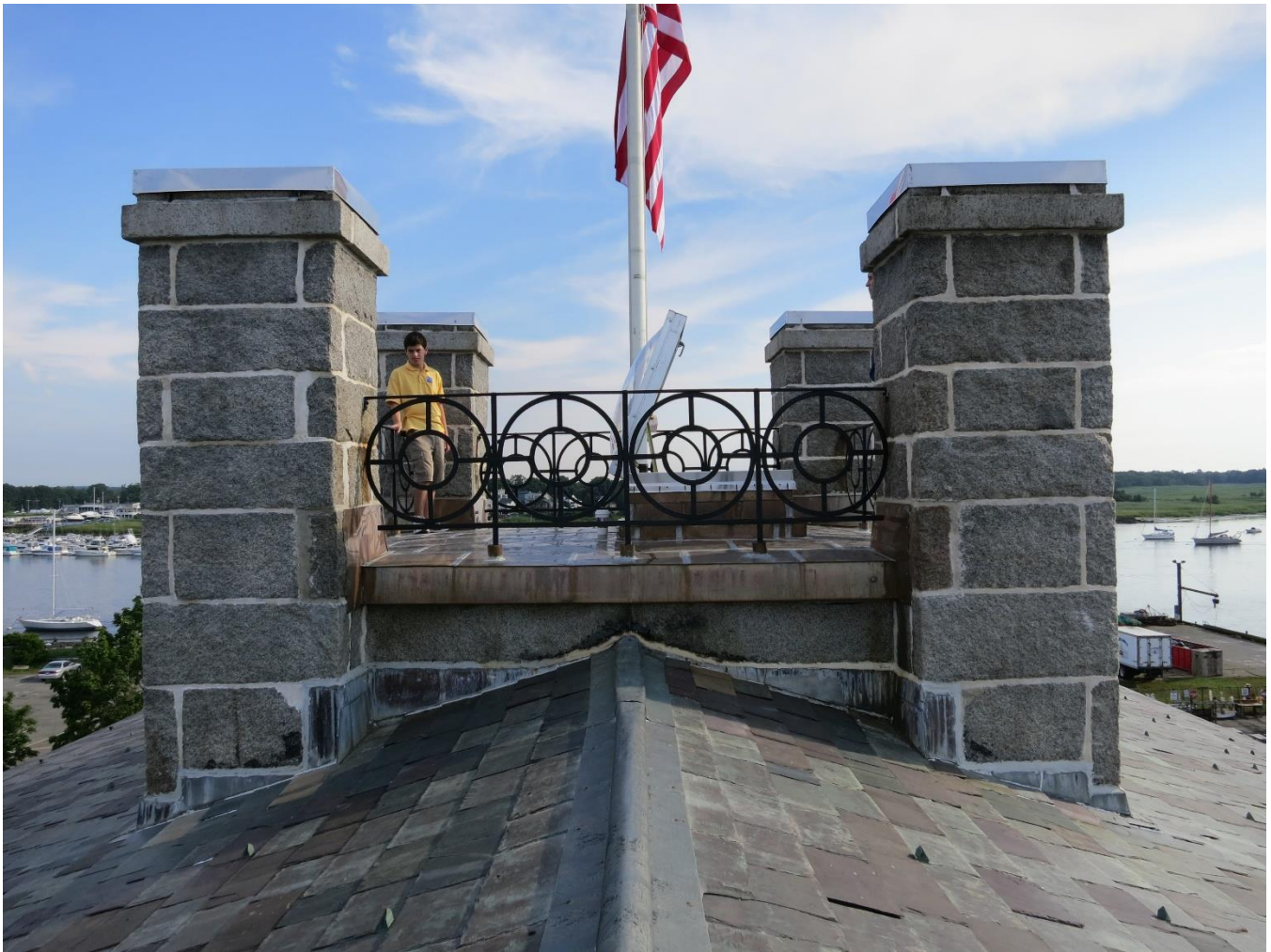
(vi) 7/24/2013 Observatory guardrail detail, Gregory Colling
