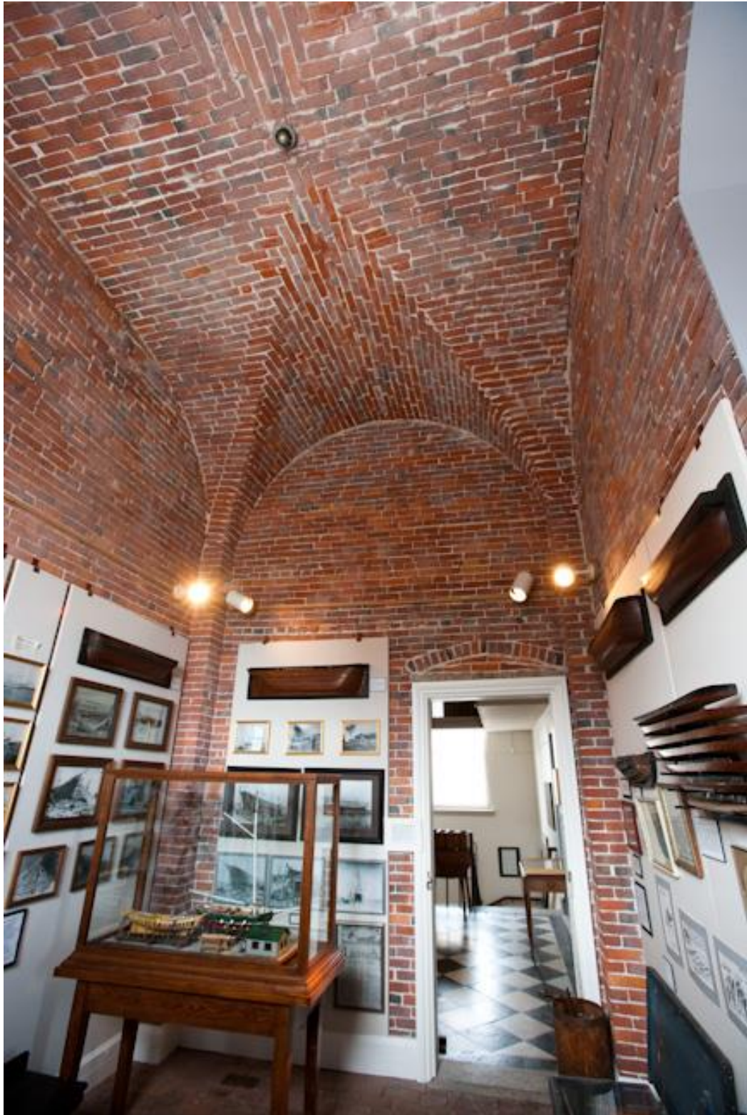
(ix) 6/2/2009 Second floor groin vault (Baker Gallery), Carl Tremblay
