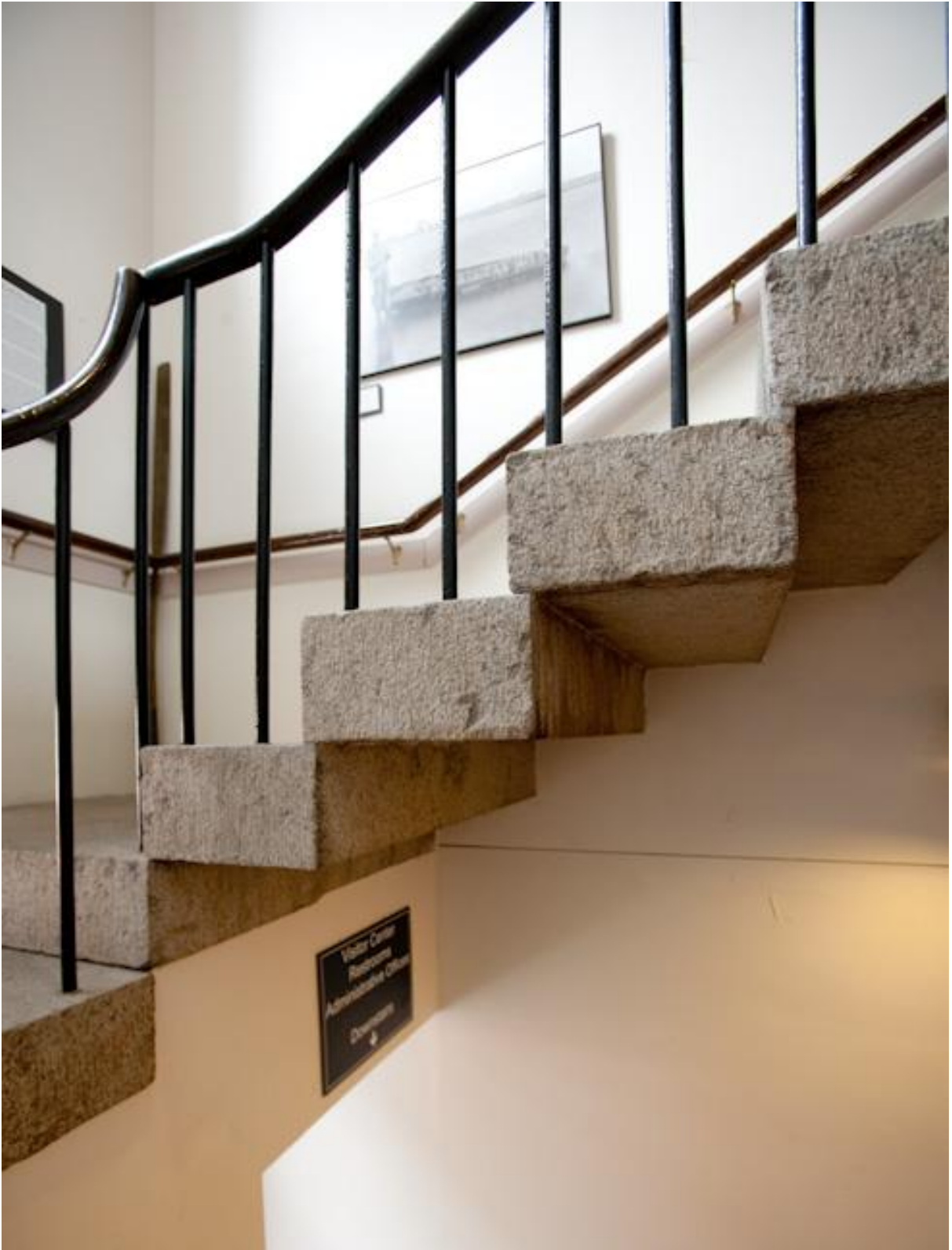
(viii) 6/2/2009 Interior Hanging Stair Detail, Carl Tremblay
