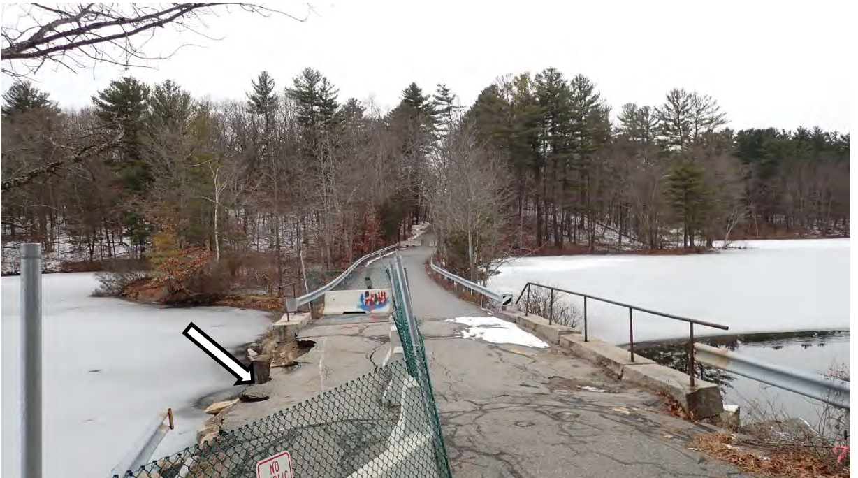
Photo #2: View northwest of Plummer Spring Rd, Newburyport facing Middle St, West Newbury over the Upper Artichoke Reservoir. Arrow indicates the failed section at the southern end of the roadway, directly over the bridge which is closed for public safety.
