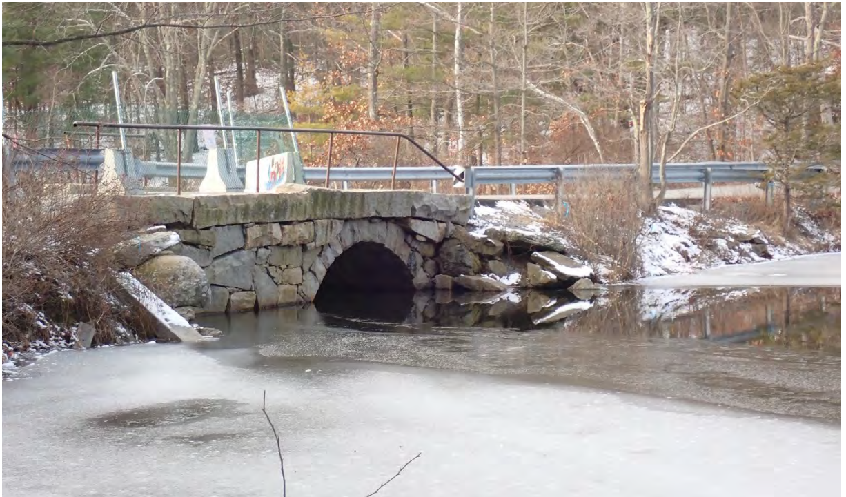
Photo #6: View southwest of the northern side of the roadway and bridge over the Upper Artichoke Reservoir.
