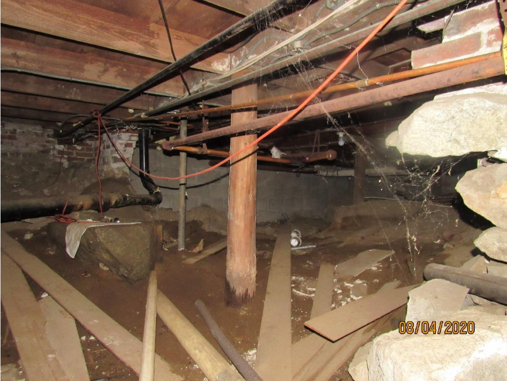
Photo 7 Antiquated timber framing with posts extending below grade and foundation walls demolished
