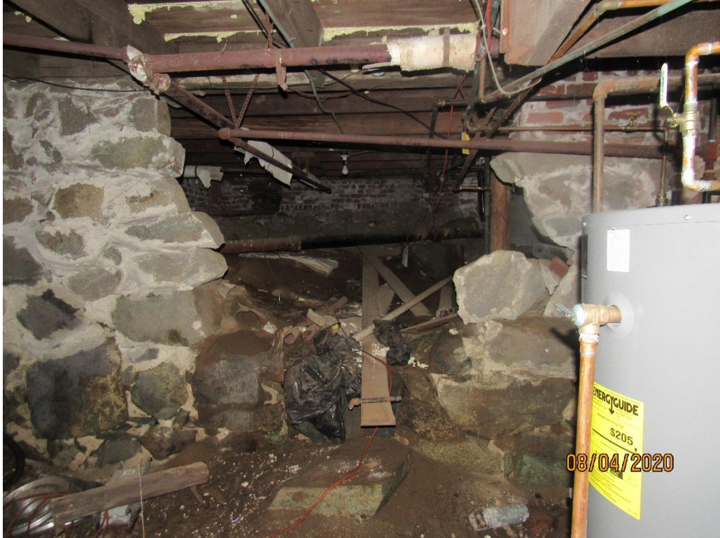
Photo 8 Foundation walls partially demolished to allow additions
