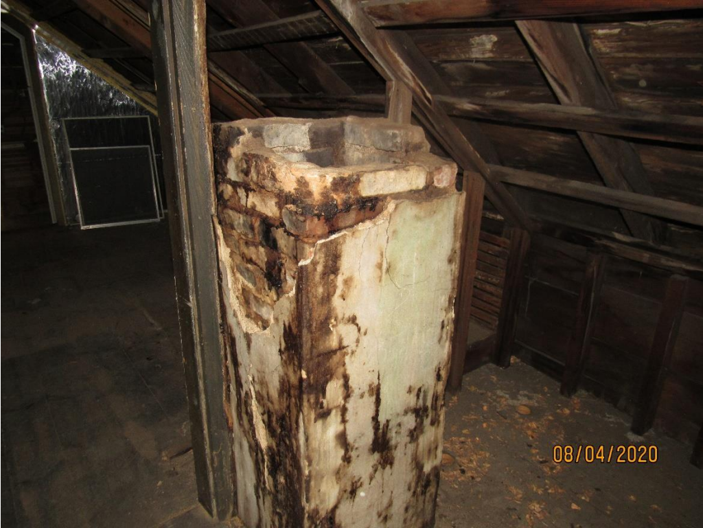
Photo 9 Balloon framed walls to support roof and chimney demolished and abandoned in the attic
