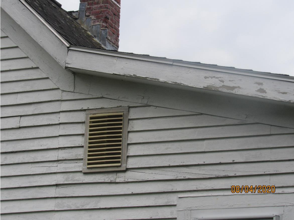
Photo 11 Ventilation beneath the roof
