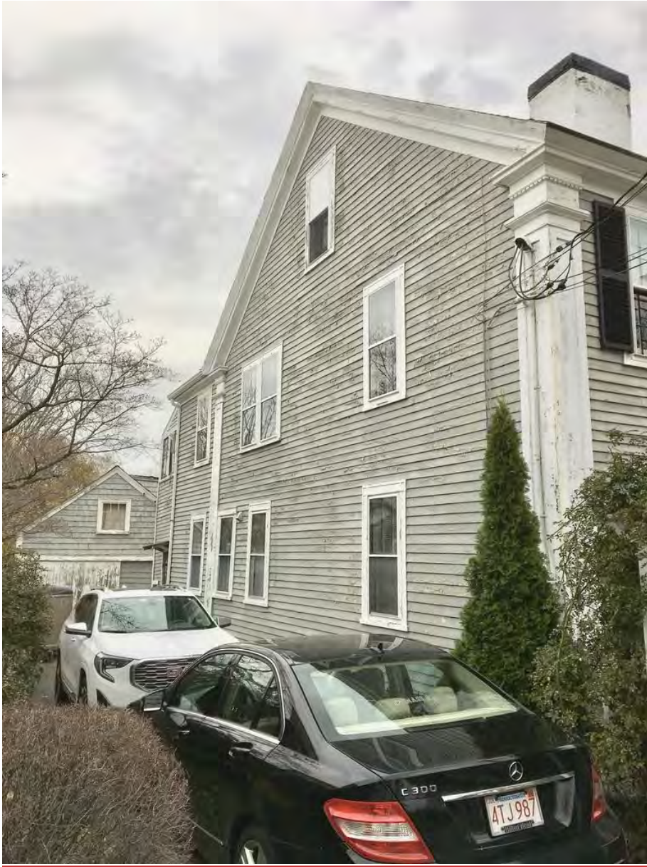
7. West Façade – Corner Pilaster, Window Trim, Rake Detail
