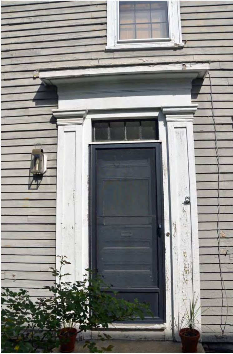
12. East Entry Door with Transom Window, Pilasters, Frieze, and Cornice Detail.
