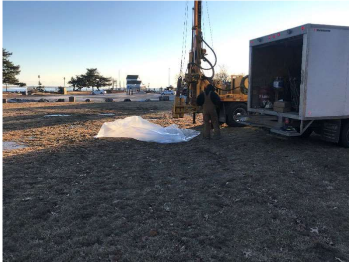
Photo 1 - View of NEBC preparing to drill NB-3
