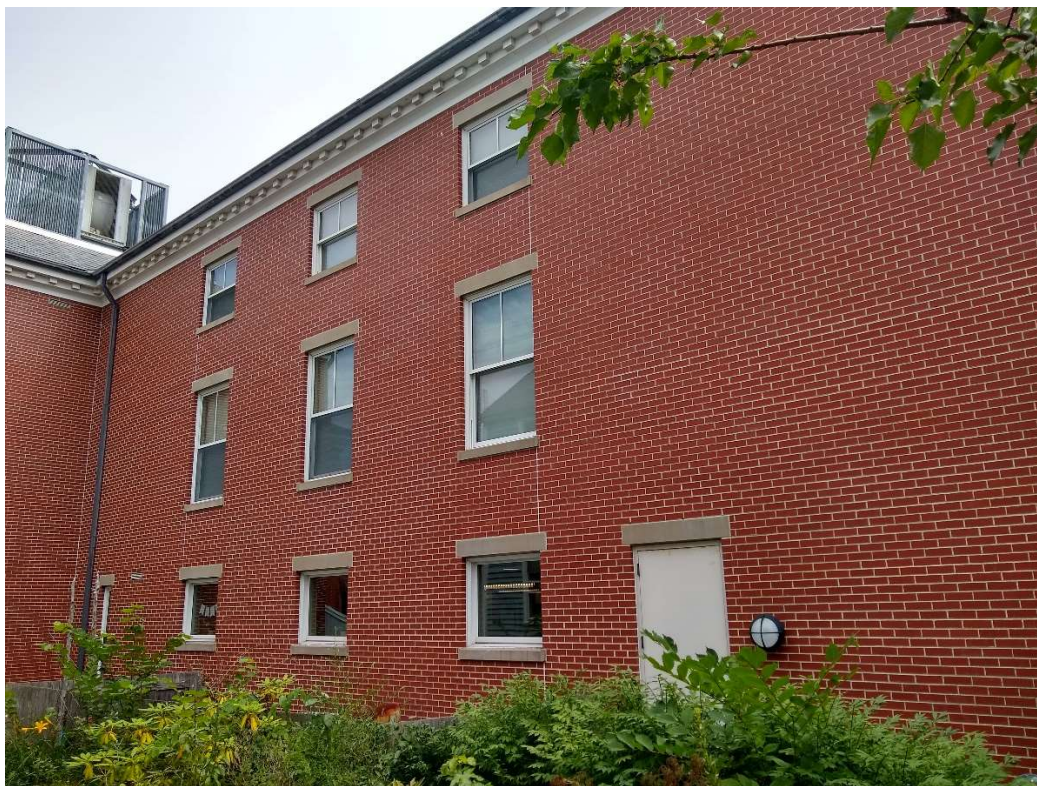
Photo No. 6: Molin Wing – West Façade (August 2020)
