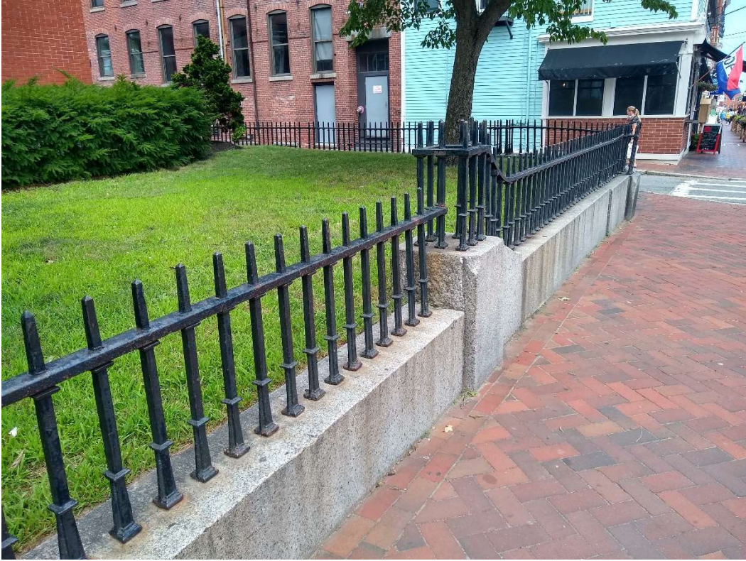
Photo No. 14: Tracy Mansion Fence – East Façade (August 2020)
