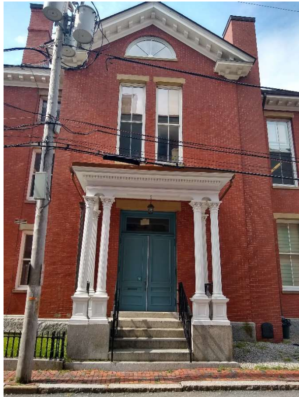
Photo No. 13: Simpson Annex Portico (August 2020)
