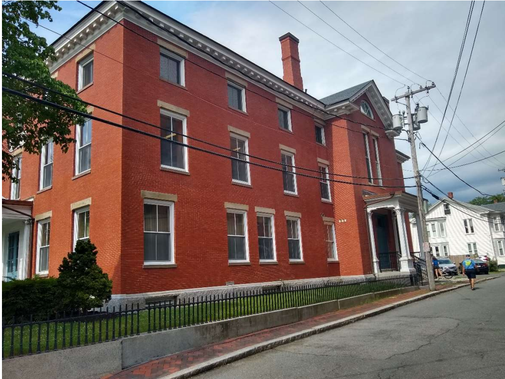
Photo No. 2: Tracy Mansion – North Façade (July 2020)
