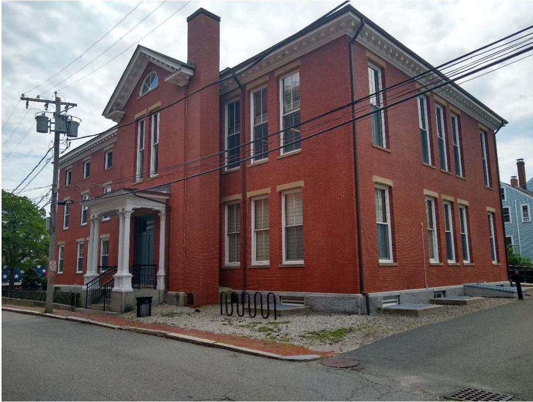
Photo No. 3: Simpson Annex – North Façade (August 2020)
