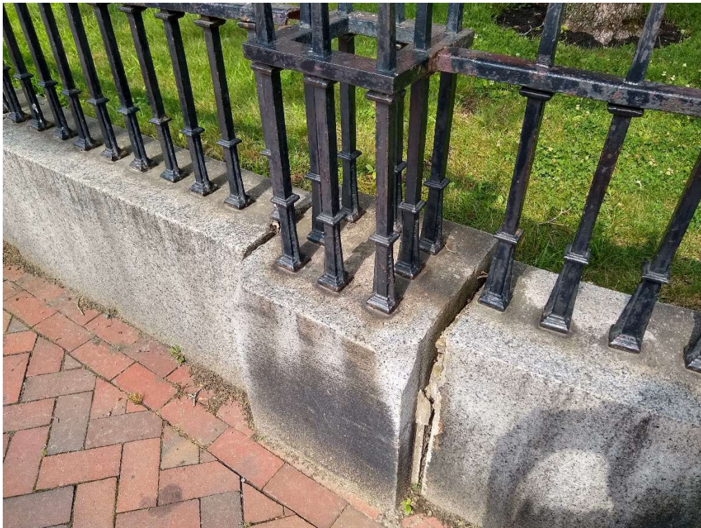
Photo No. 15: Tracy Mansion Fence – Detail (August 2020)
