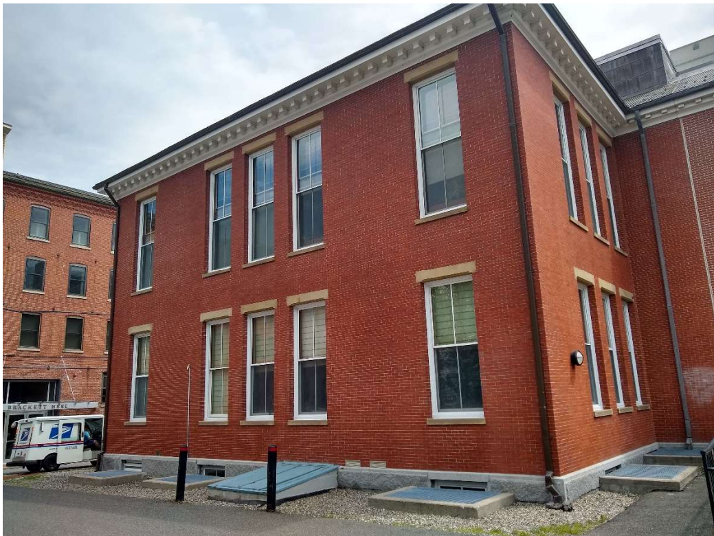
Photo No. 4: Simpson Annex – West Façade (August 2020)
