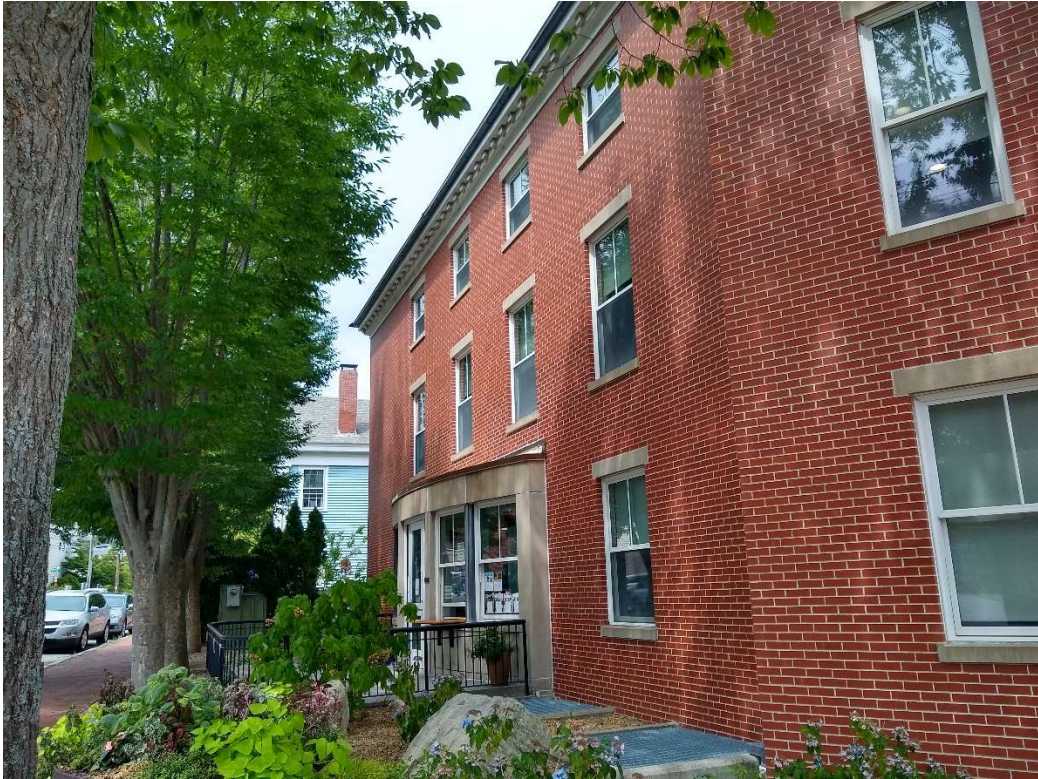
Photo No. 7: Molin Wing – South Façade (August 2020)
