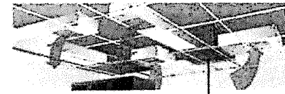
5-Ton Ducted Liebert Mini-Mate2
