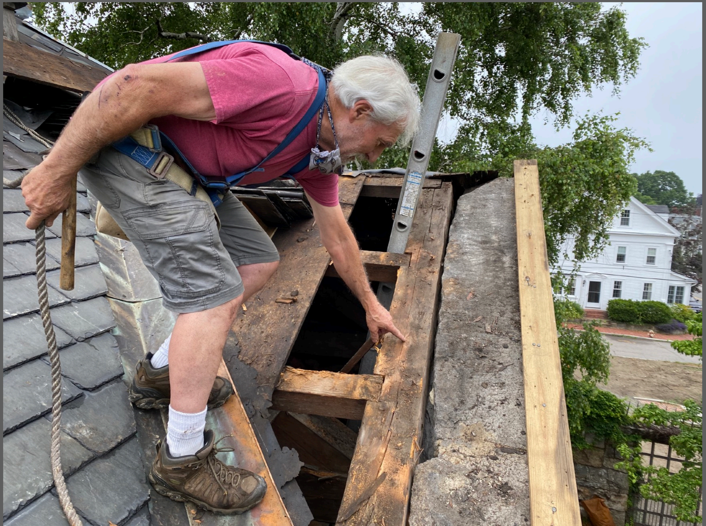
ROOF OPENED TO ATTIC WARREN SOULARD SLATE ROOFER
