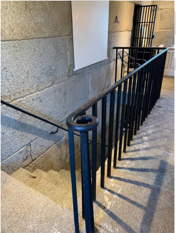
Iron Handrail and Baluster
