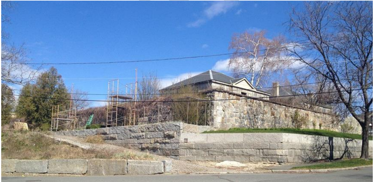
Granite Low Walls
