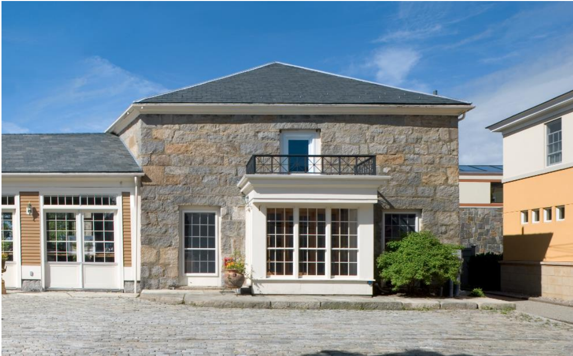
Auburn Street Façade
