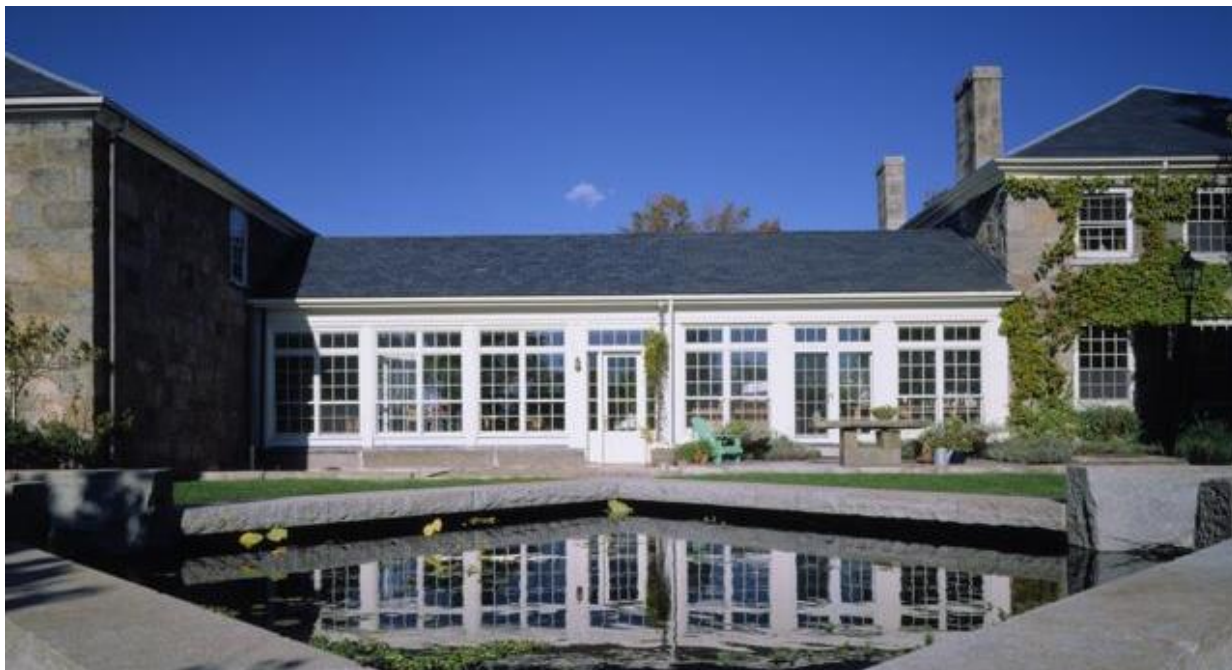
Non-Contributing Connector Building
