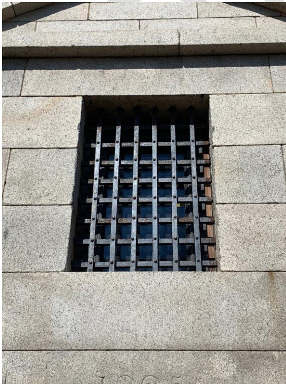
Auburn Street Hallway Window
