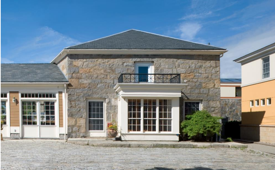
Auburn Street Façade
