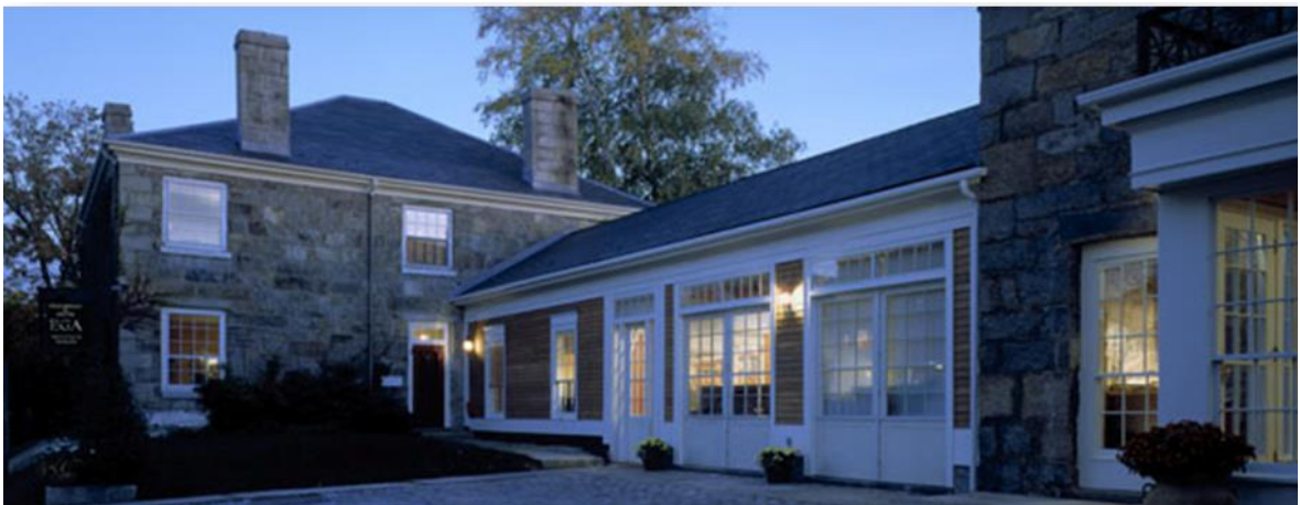
Vernon Street Frontage
