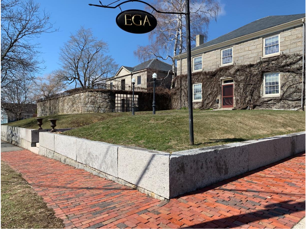
Auburn Street Frontage Walls
