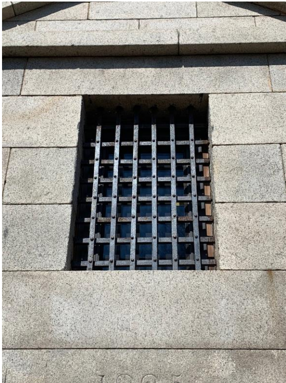
Auburn Street Hallway Window
