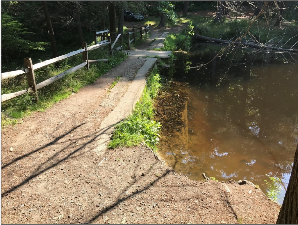
Photograph 1: Upstream side of Flowering Pond Dam.
