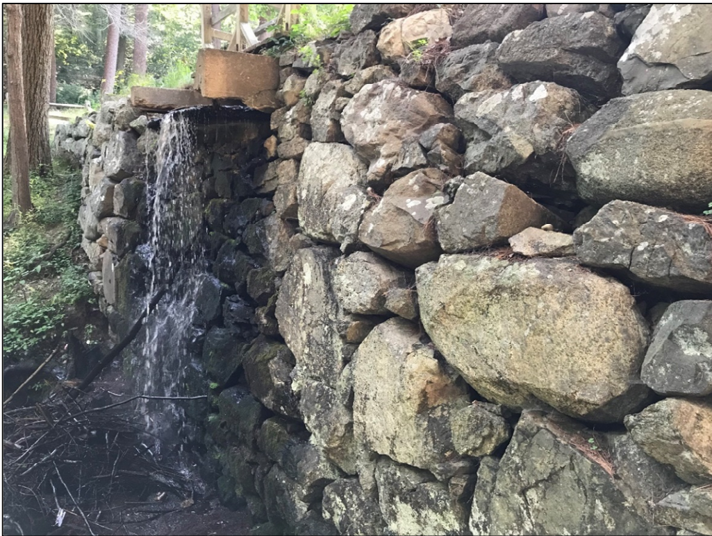
Photograph 2: Downstream side of Flowering Pond Dam.
