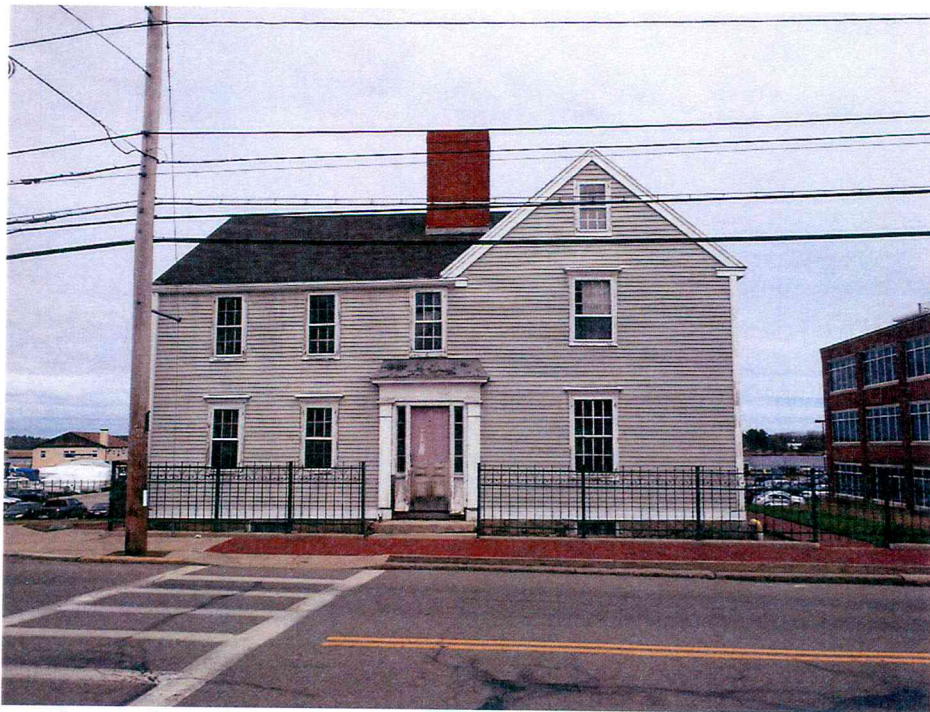
3. Street (west) elevation – April 2015
