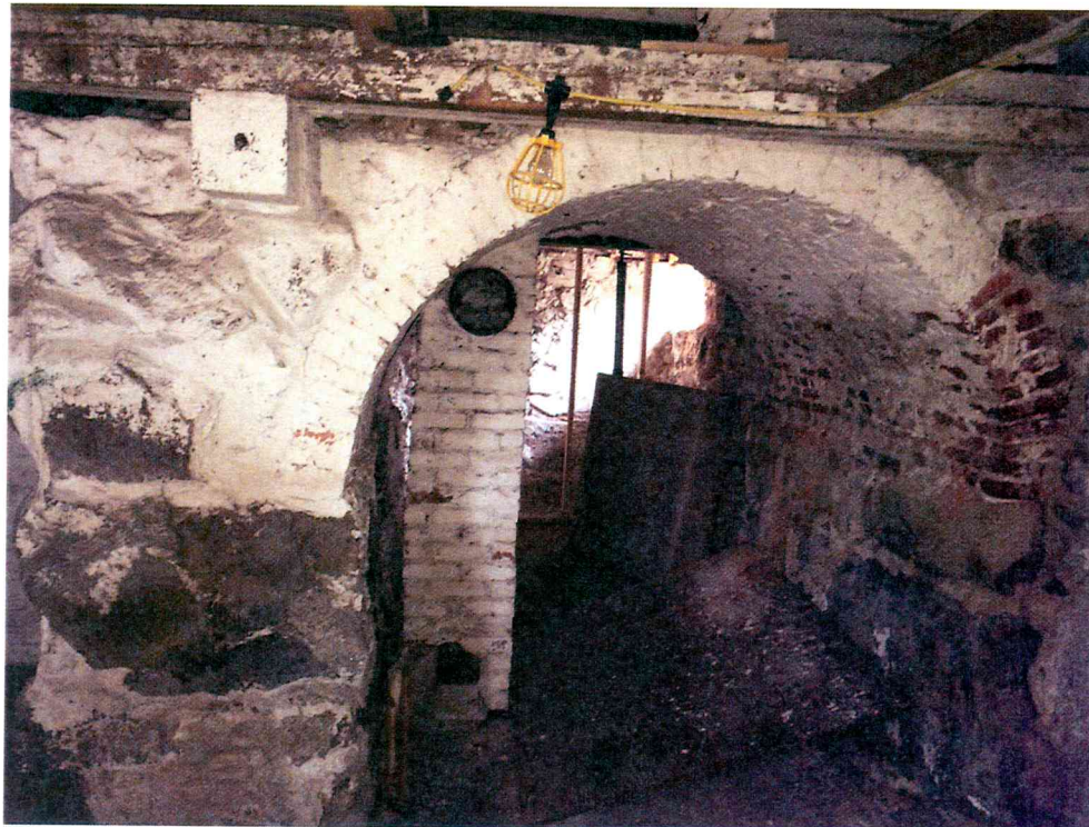
9. Basement arch and foundation – June 2015
