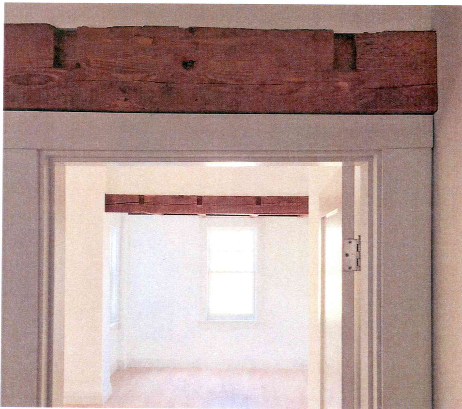
14. Exposed beams at second floor master bedroom – March 2017
