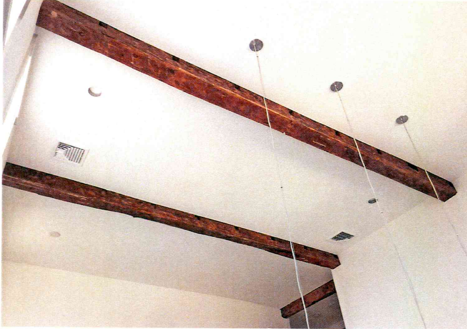
13. Exposed second floor beams – March 2017
