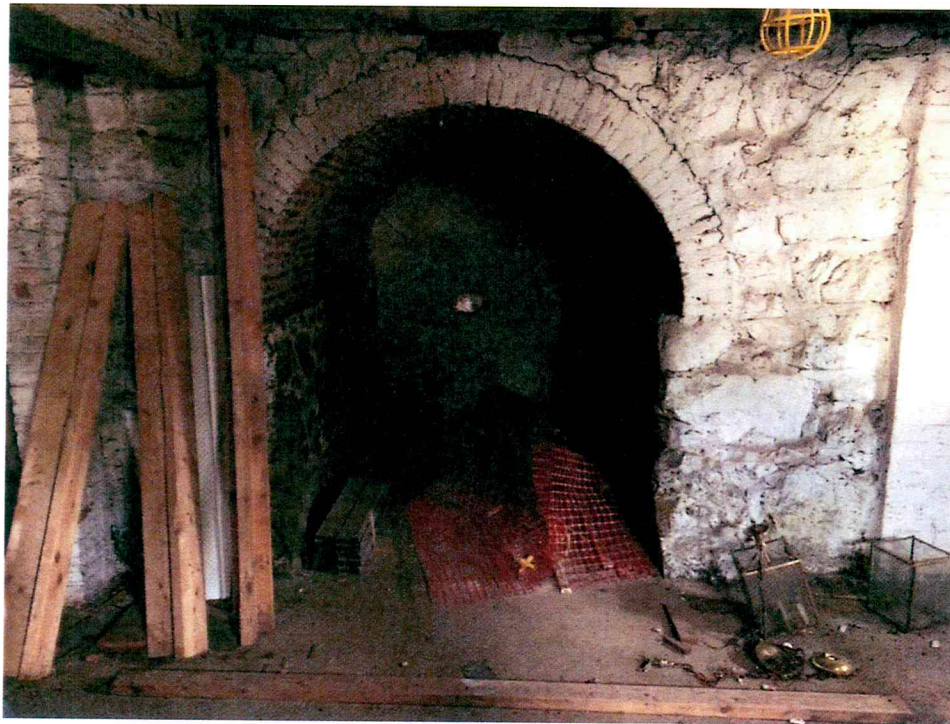
7. Basement arch and foundation – June 2015
