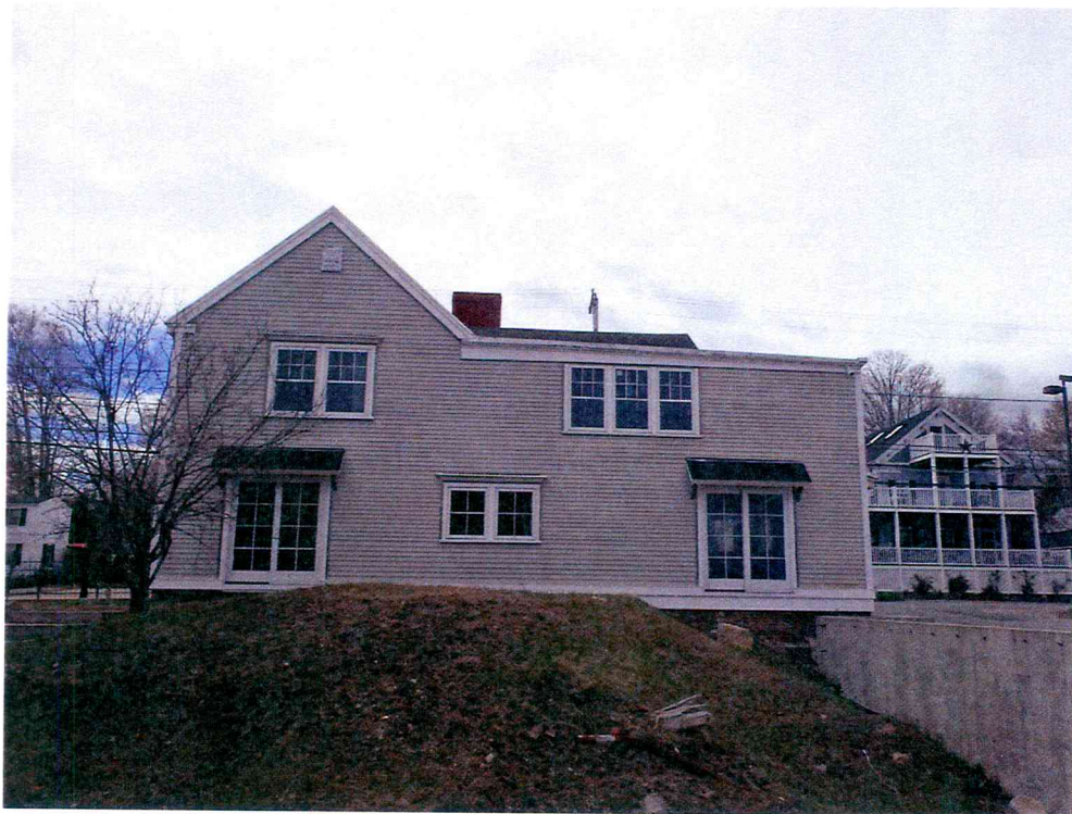
5. Rear (east) elevation – April 2015
