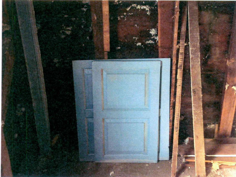
12. Interior shutters for window on second floor, street (west) elevation – March 2016
