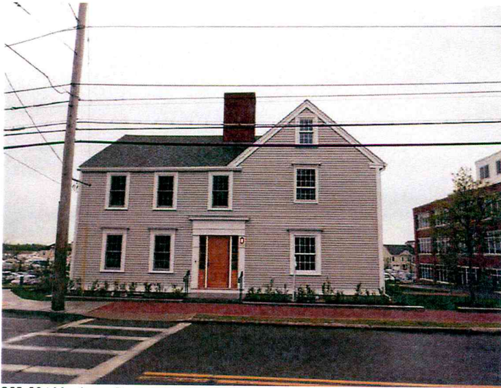
262-264 Merrimac Street, camera facing northeast
