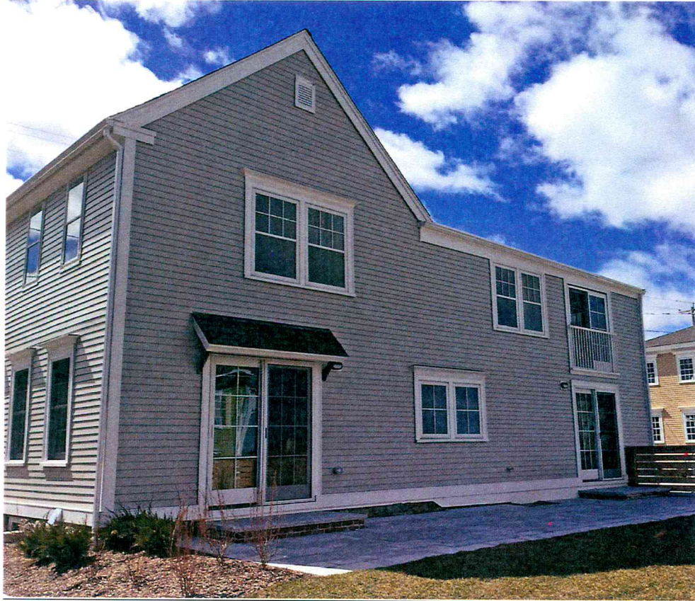
18. Rear (east) elevation – April 2017
