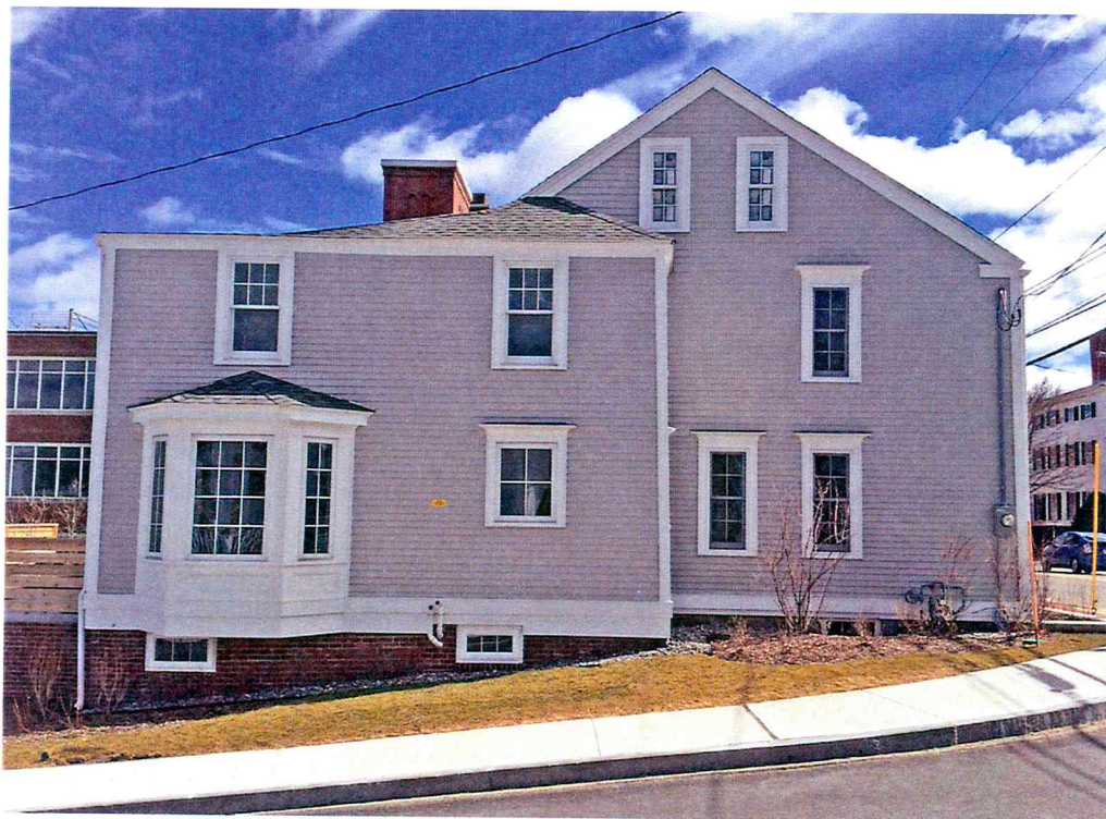
17. Left (north) elevation – April 2017
