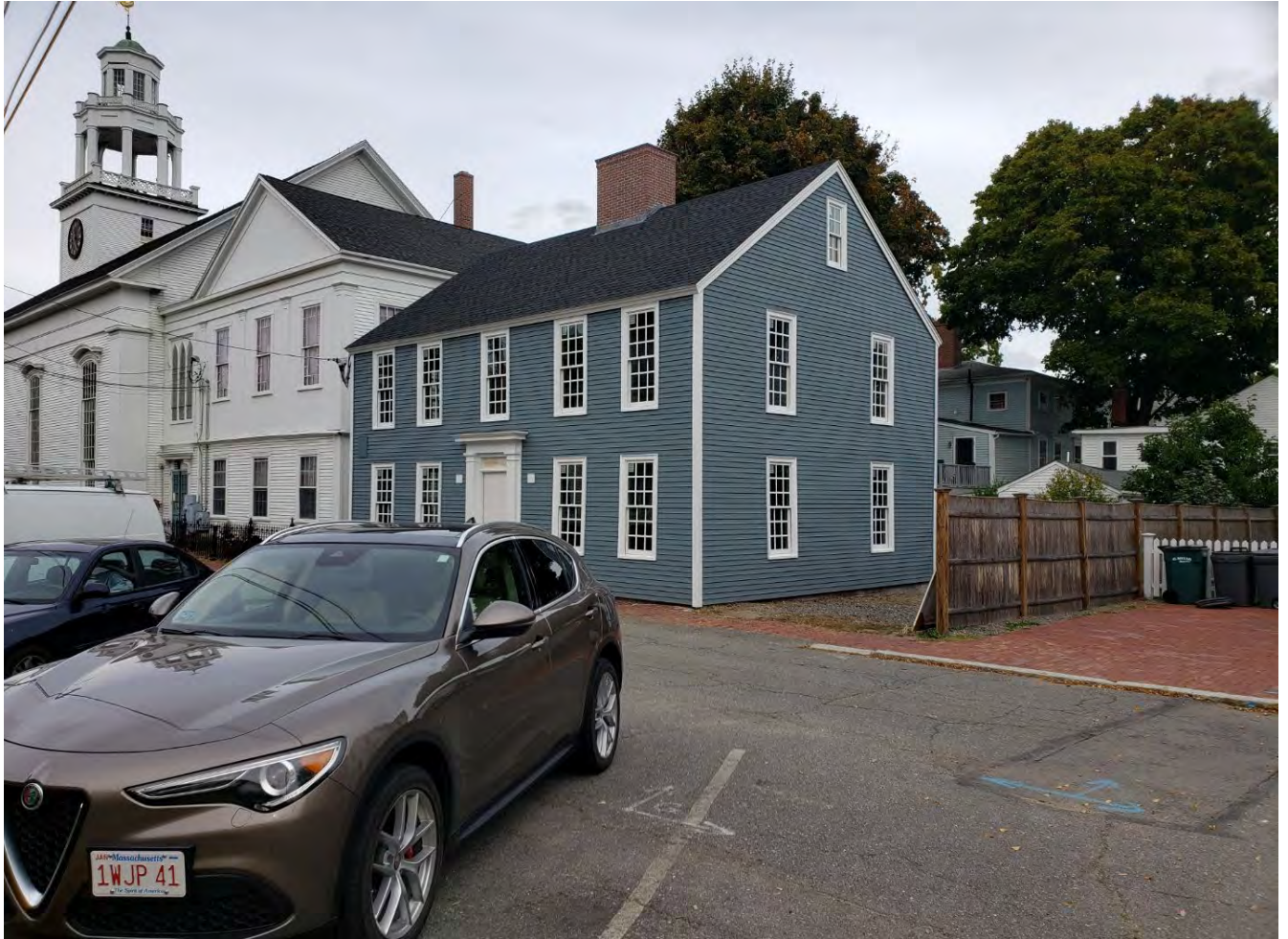
3-5 School Street after renovation
