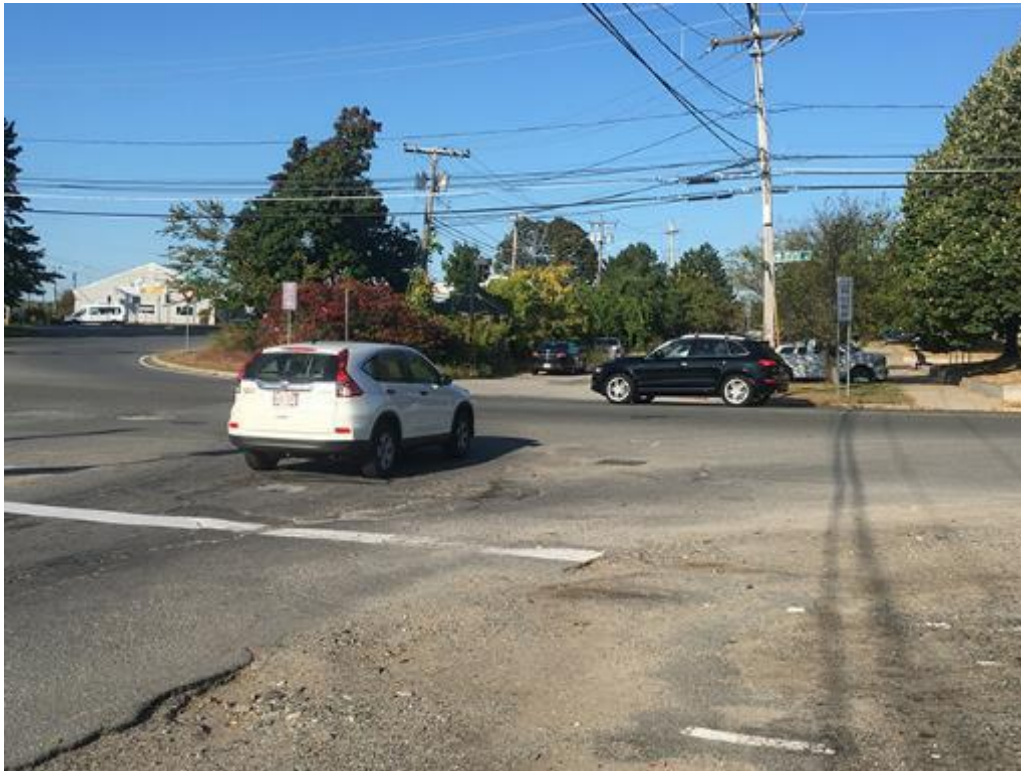
West across State St/Parker St intersection: no crosswalk or pedestrian & bicyclist accommodations
