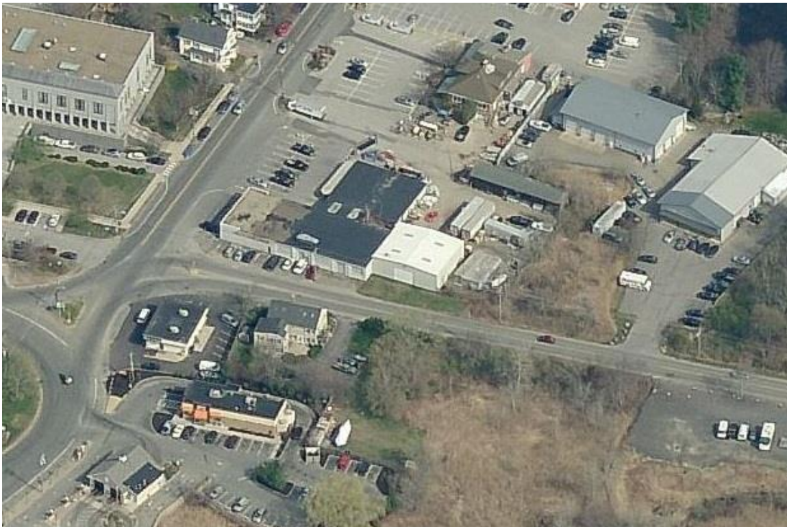
Aerial view of project area: State St/Parker St intersection and Parker Street
