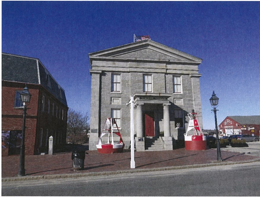
1. 3/18/2019 South building façade
