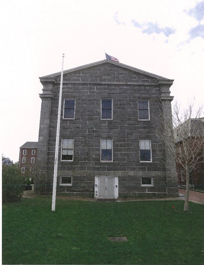
9. 5/6/2020 North Building Facade
