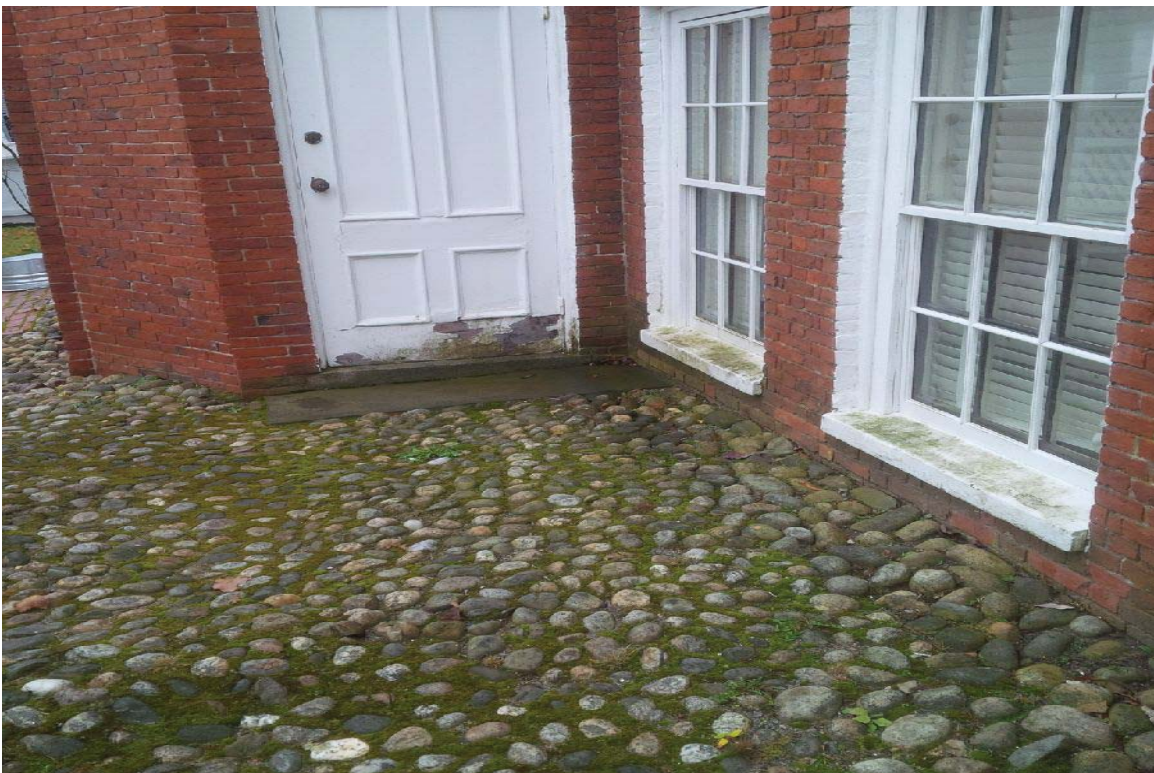
CY6: Close up of Cushing House East entrance
