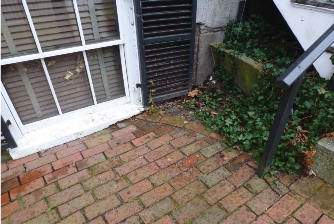
SY7: Detail of window by staircase threshold on side yard
