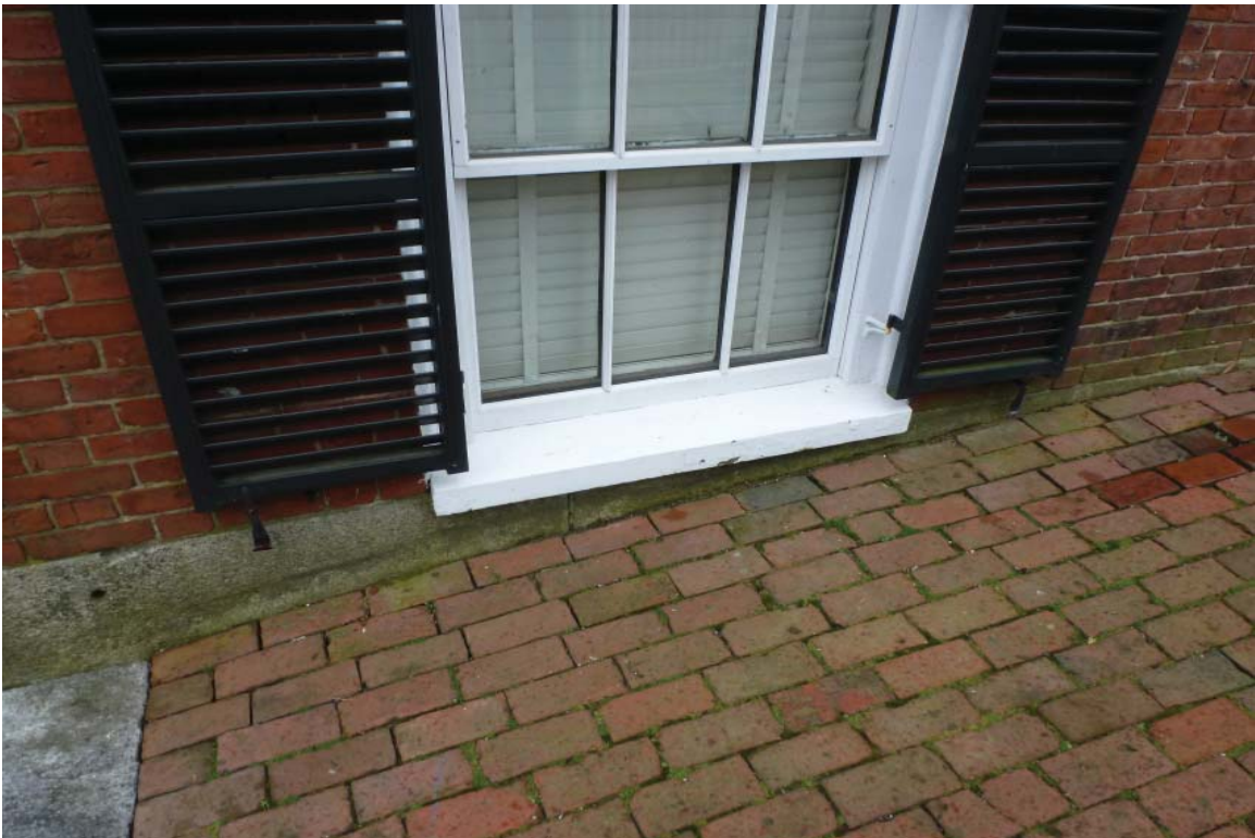
SY6: Detail of windowsill along side yard
