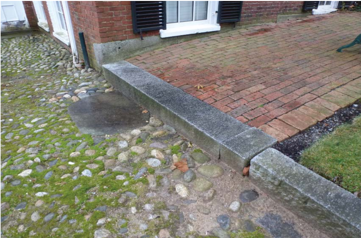
CY9: Close up of granite curb and step on Side Yard path
