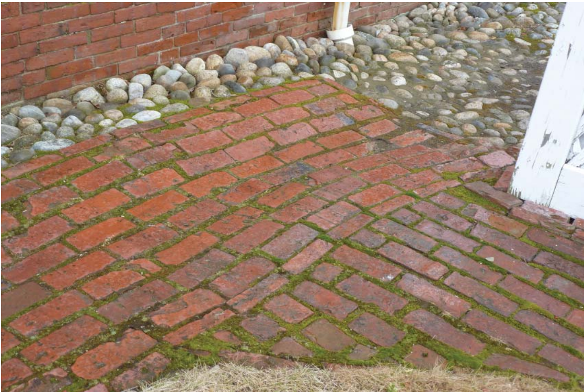
LY9: Detail of brick walkway leading from Courtyard toward Laundry Yard
