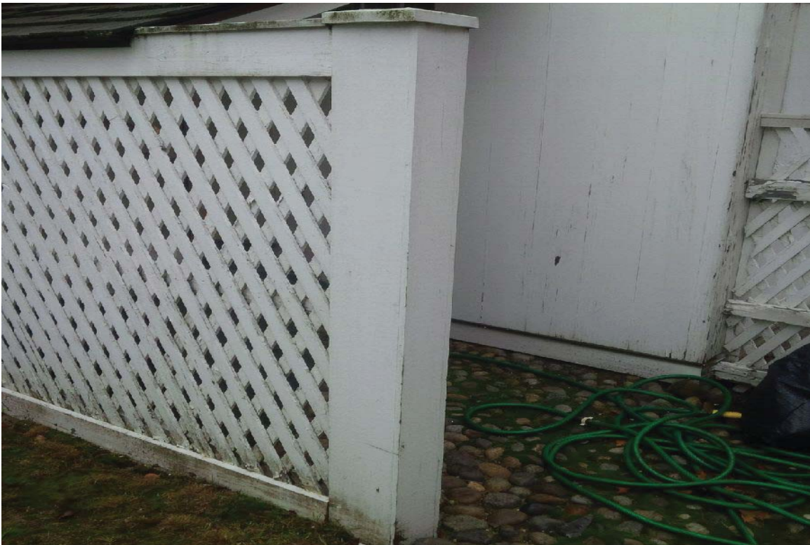
CY16: Close up view of fence enclosing Laundry Shed/Privy overhang area
