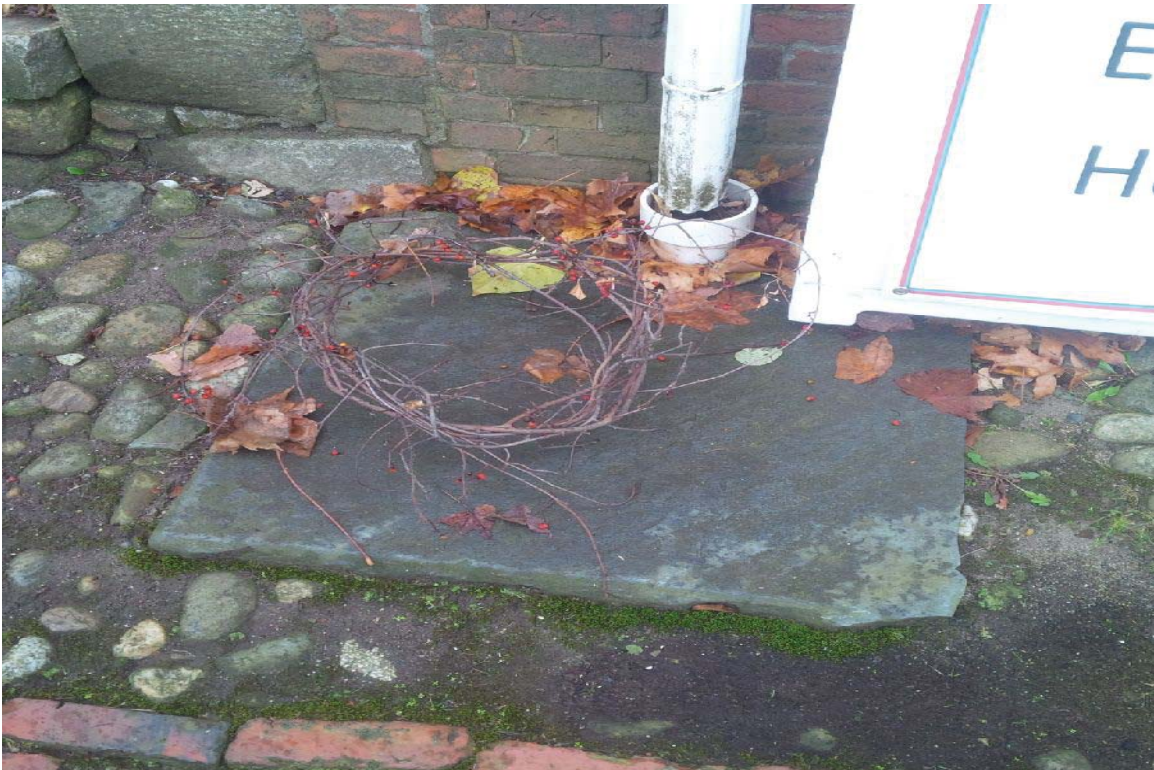
LY12: Detail view of downspout at East corner of Cushing House
