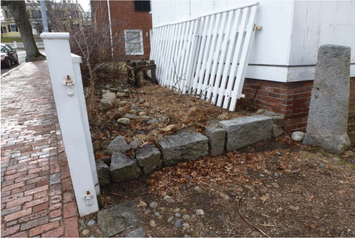
CA3: Granite edging behind Laundry Shed
