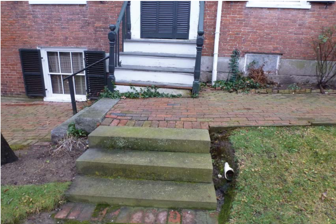
SY12: View facing Cushing House Sideyard threshold and stairs
