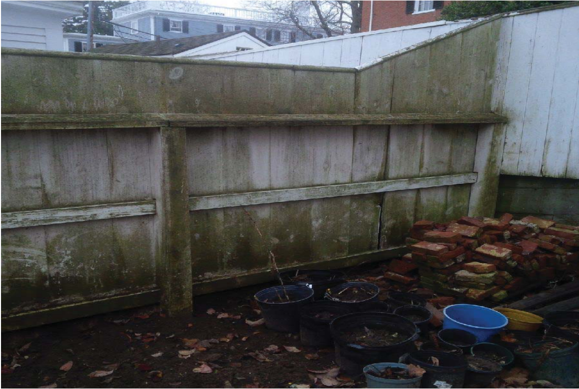
ON13: Detail of fence at Northeastern corner of Barn structure
