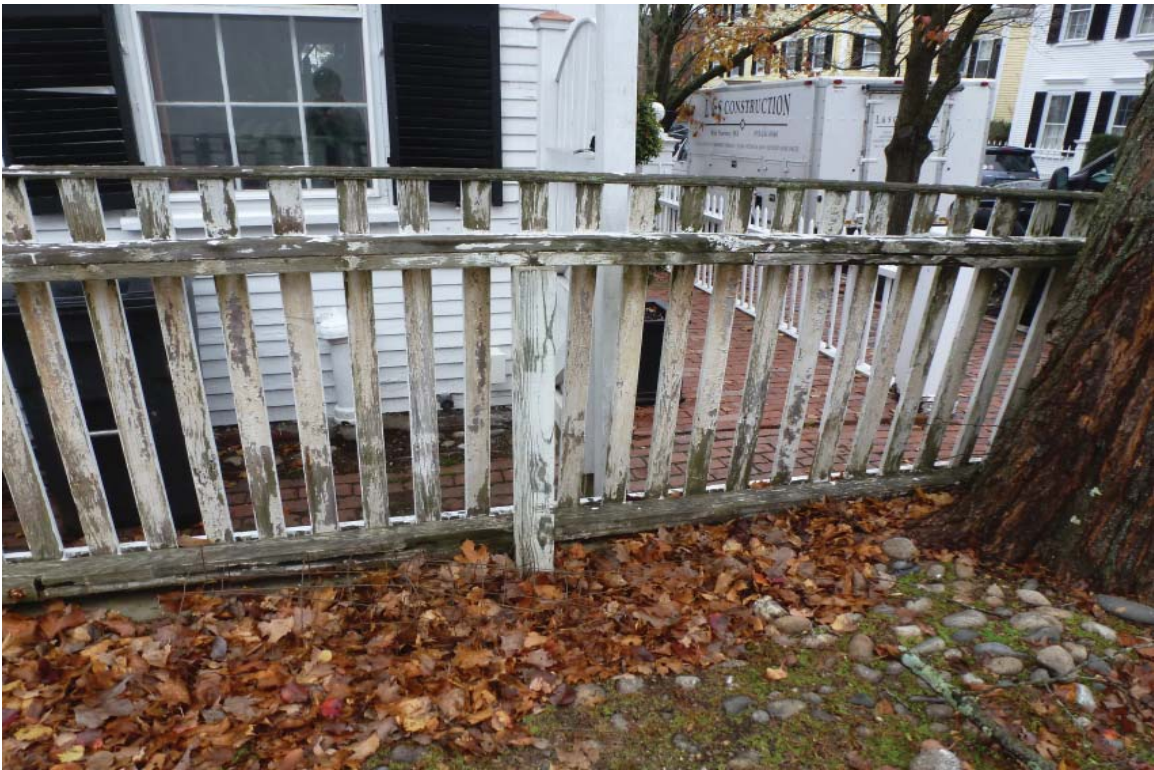
CA4: Northwest view of fence separating Cushing Alley from neighbor
