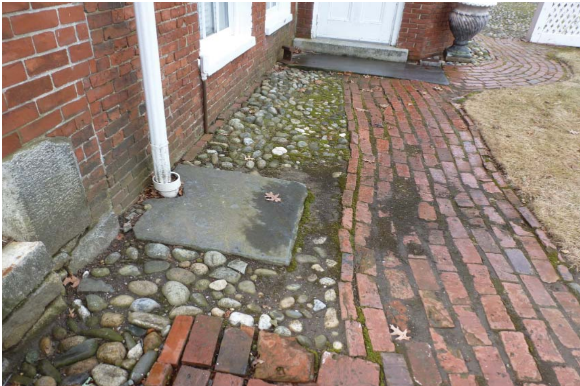
LY2: View of Cushing House Southeast lower level entryway
