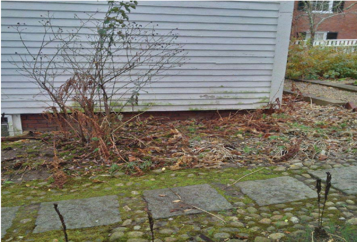
ON7: Northwest corner of Barn structure
