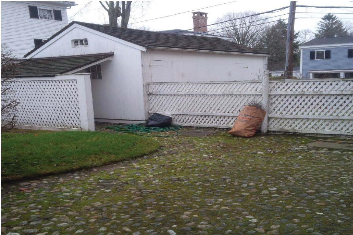
CY13: Courtyard view facing North towards Laundry Shed/Privy
