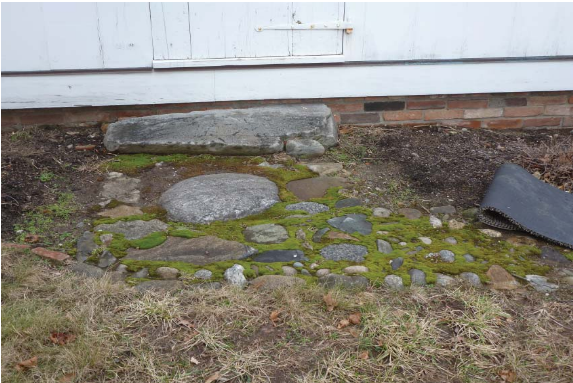
LY6: Southeastern Laundry Shed/Privy threshold
