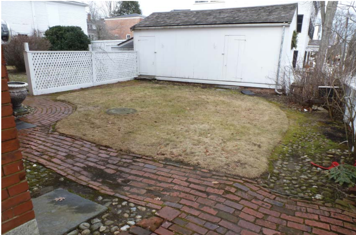
LY1: View of Laundry Yard facing North
