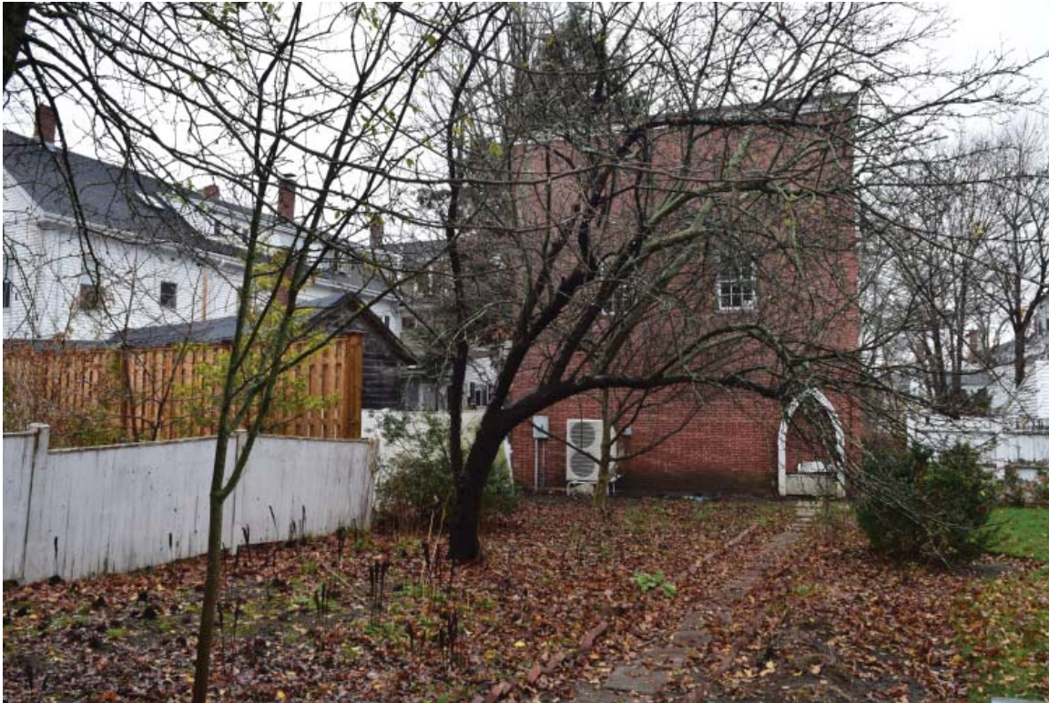
ON3: View standing from Northern Corner of Barn looking Northeast
