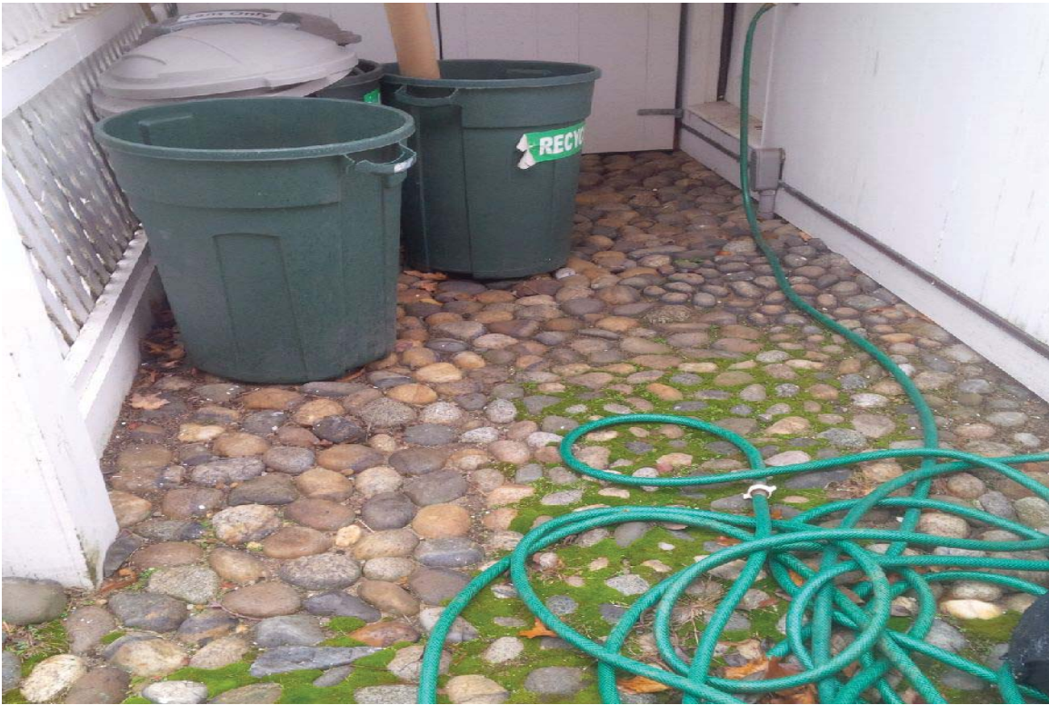
CY15: View of Laundry Shed/Privy overhang area
