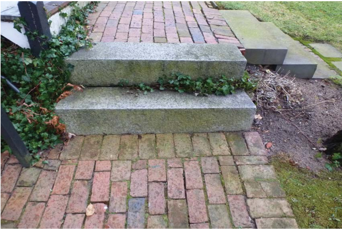
SY8: Detail of stairs leading to Cushing House sideyard threshold
