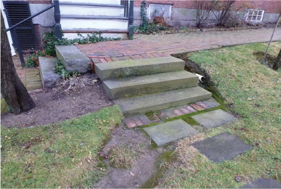
SY11: Detail of staircase at Cushing House Sideyard threshold
