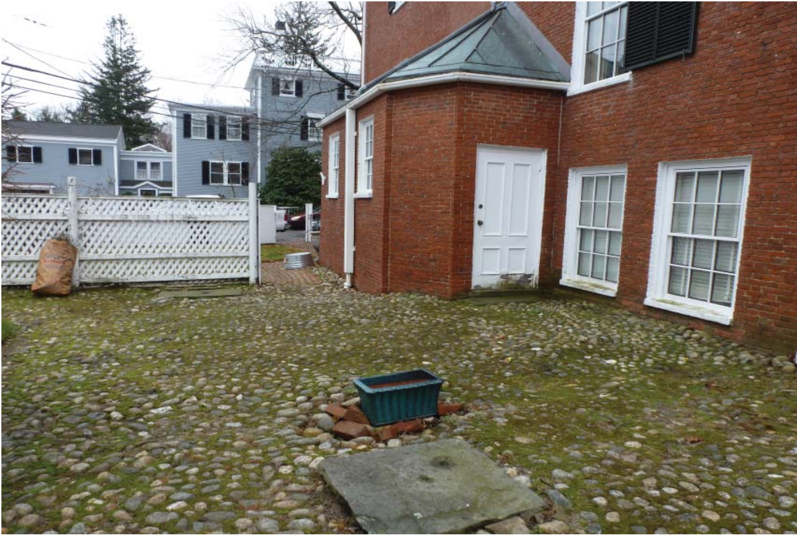
CY5: View South towards Cushing House East entrance
