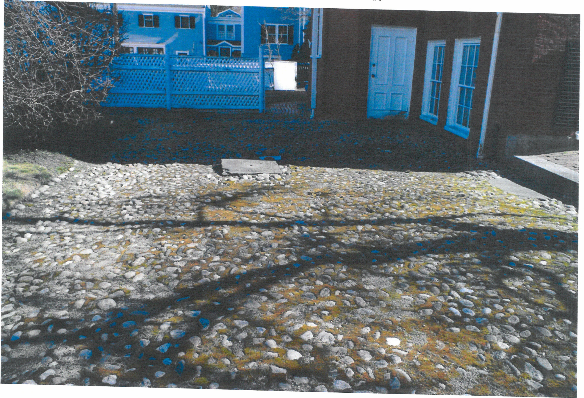
Courtyard showing uneven levels and cistern.jpg
