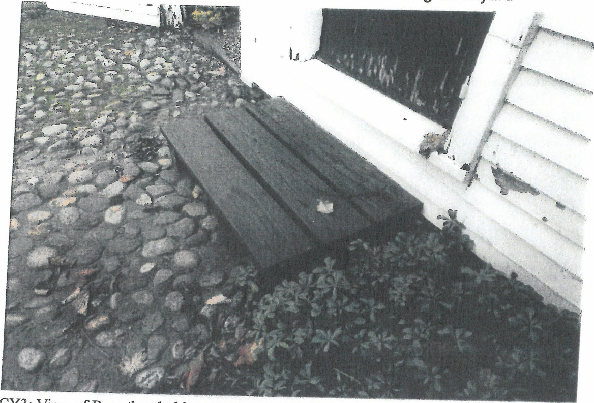
CY3: View of Barn threshold on Courtyard Side
