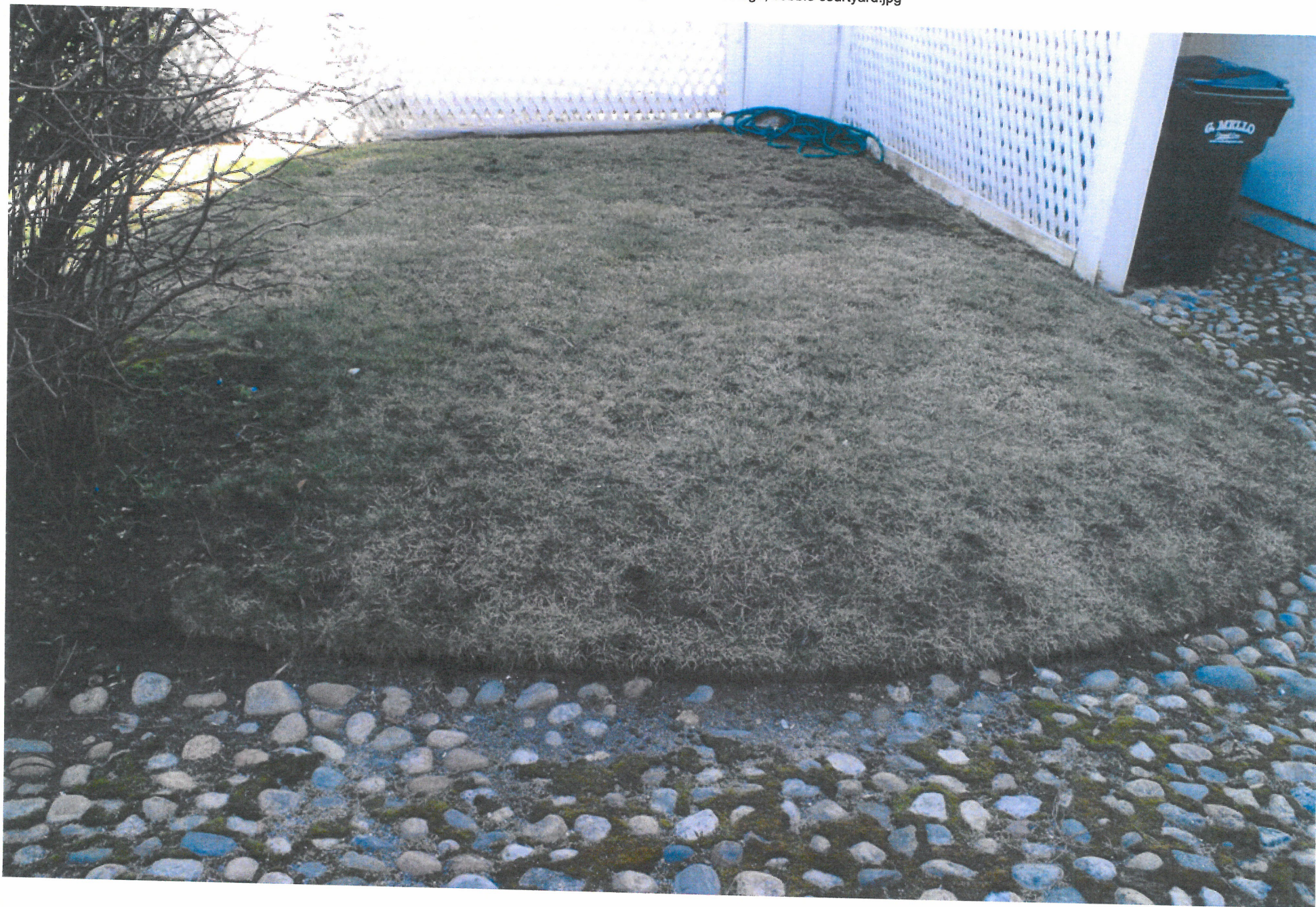
Detail of uneven grade and drainage, cobble courtyard.jpg
