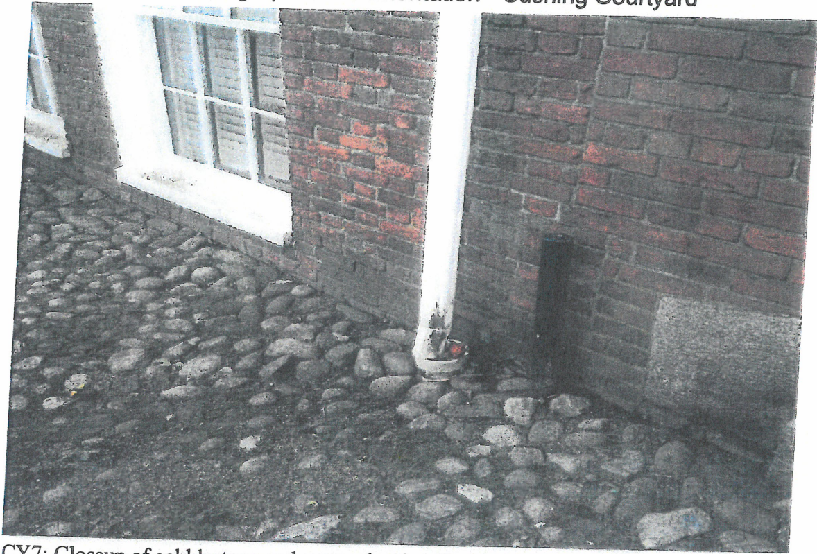
CY7: Closeup of cobblestone and gutter abutting Cushing House east side
