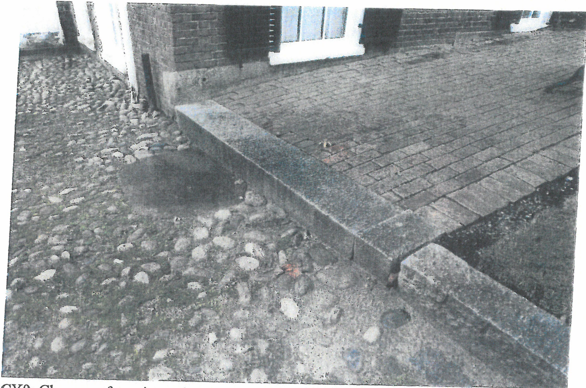
CY9: Close up of granite curb and step on Side Yard path
