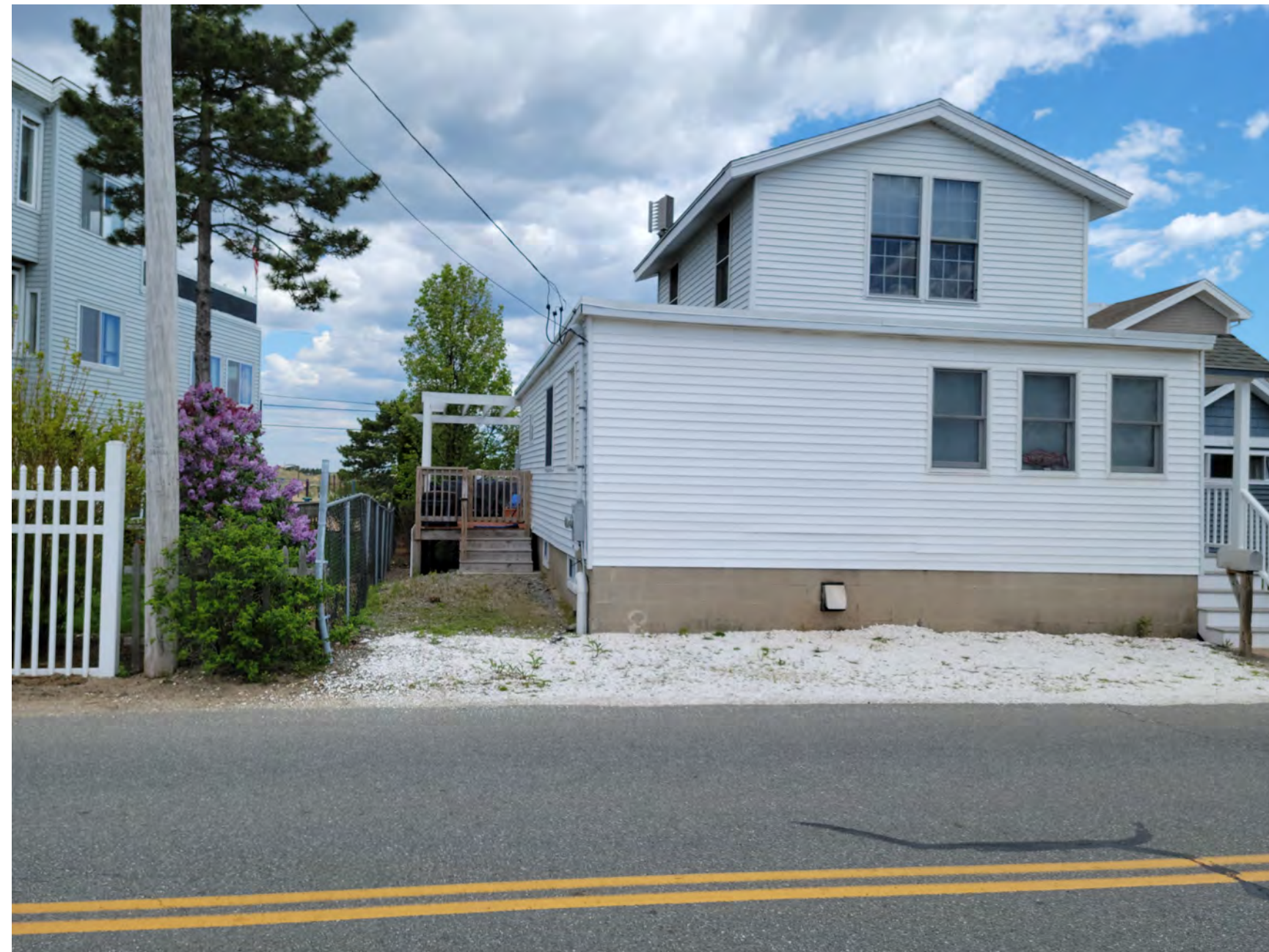
House from Northern Boulevard
