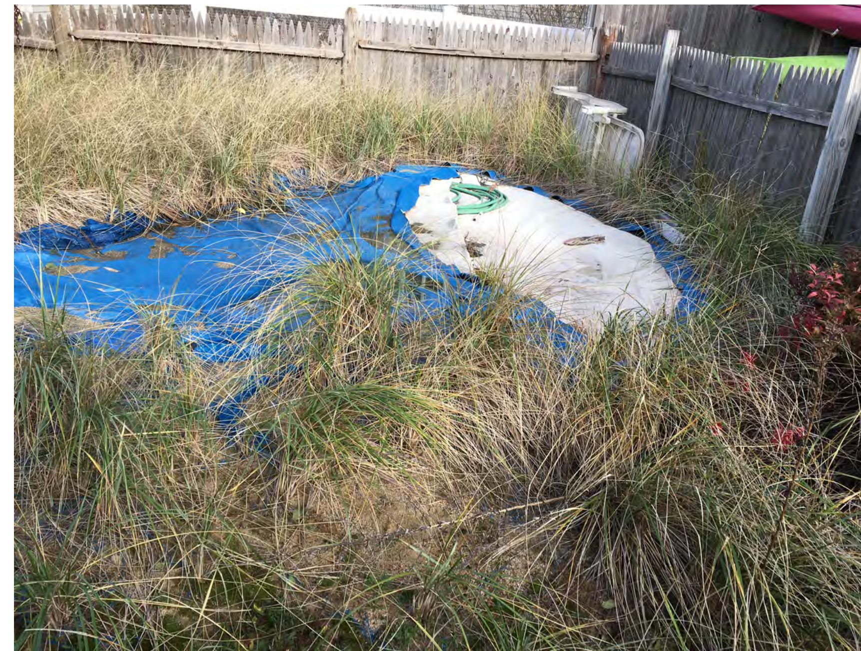
Remnants of Old Pool (liner since removed)
