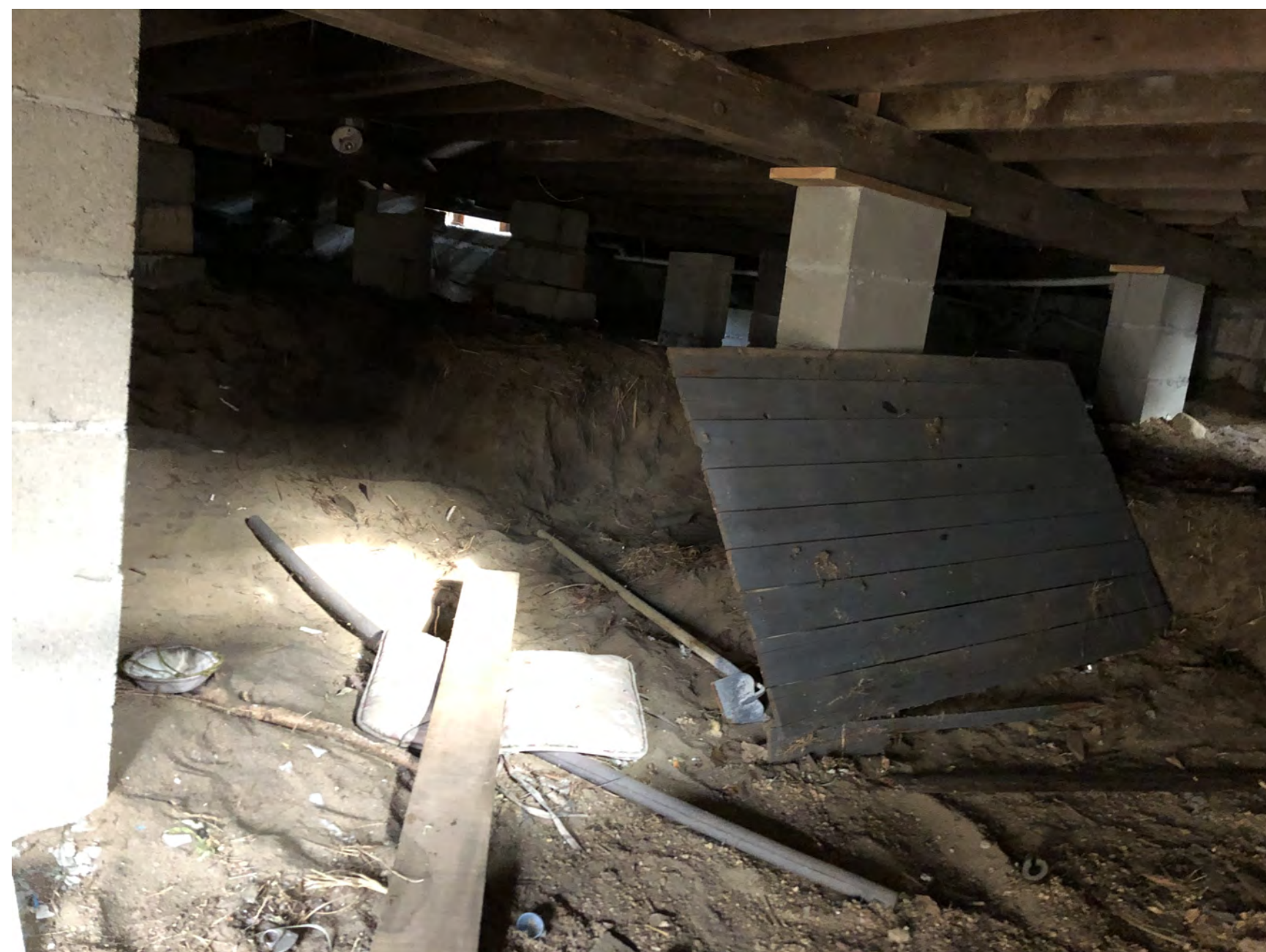
Under existing structure
