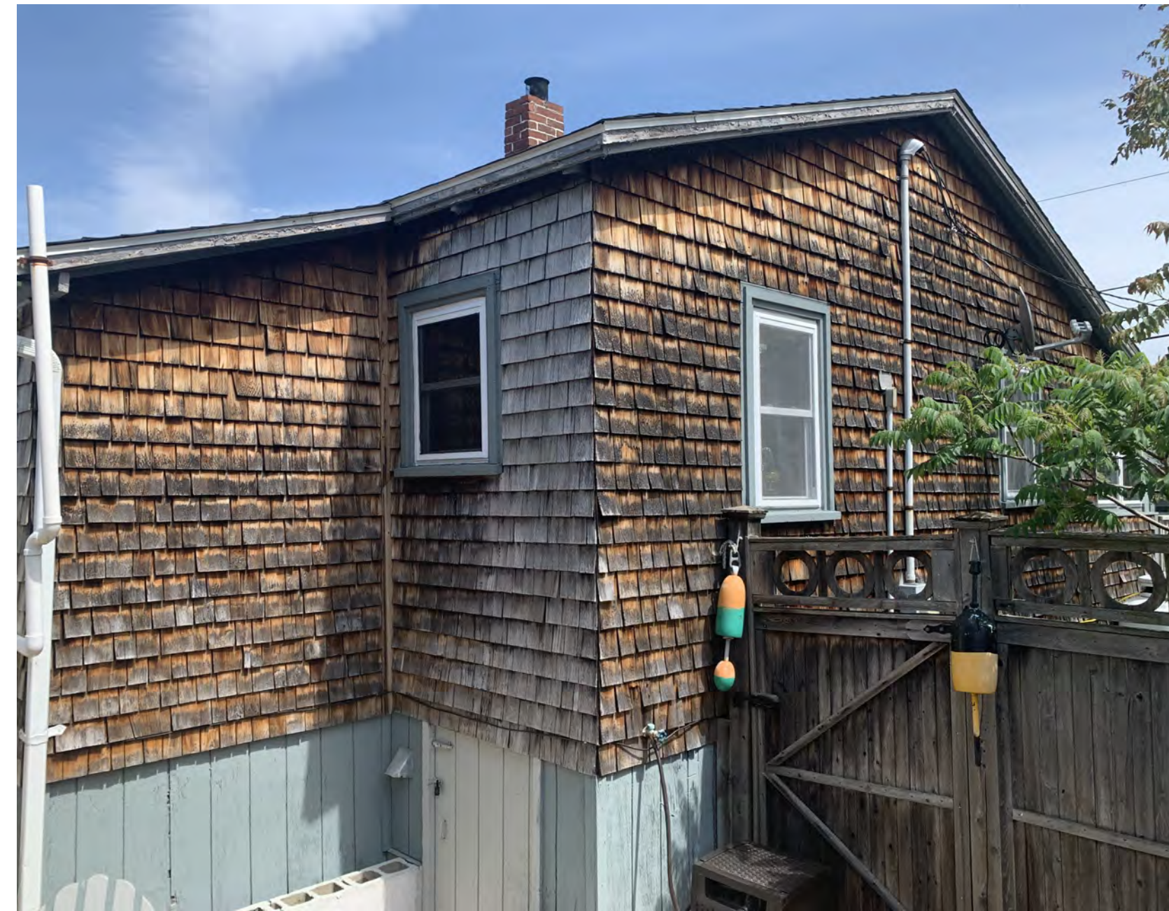
Side of house, note bottom enclosed and solid fence
