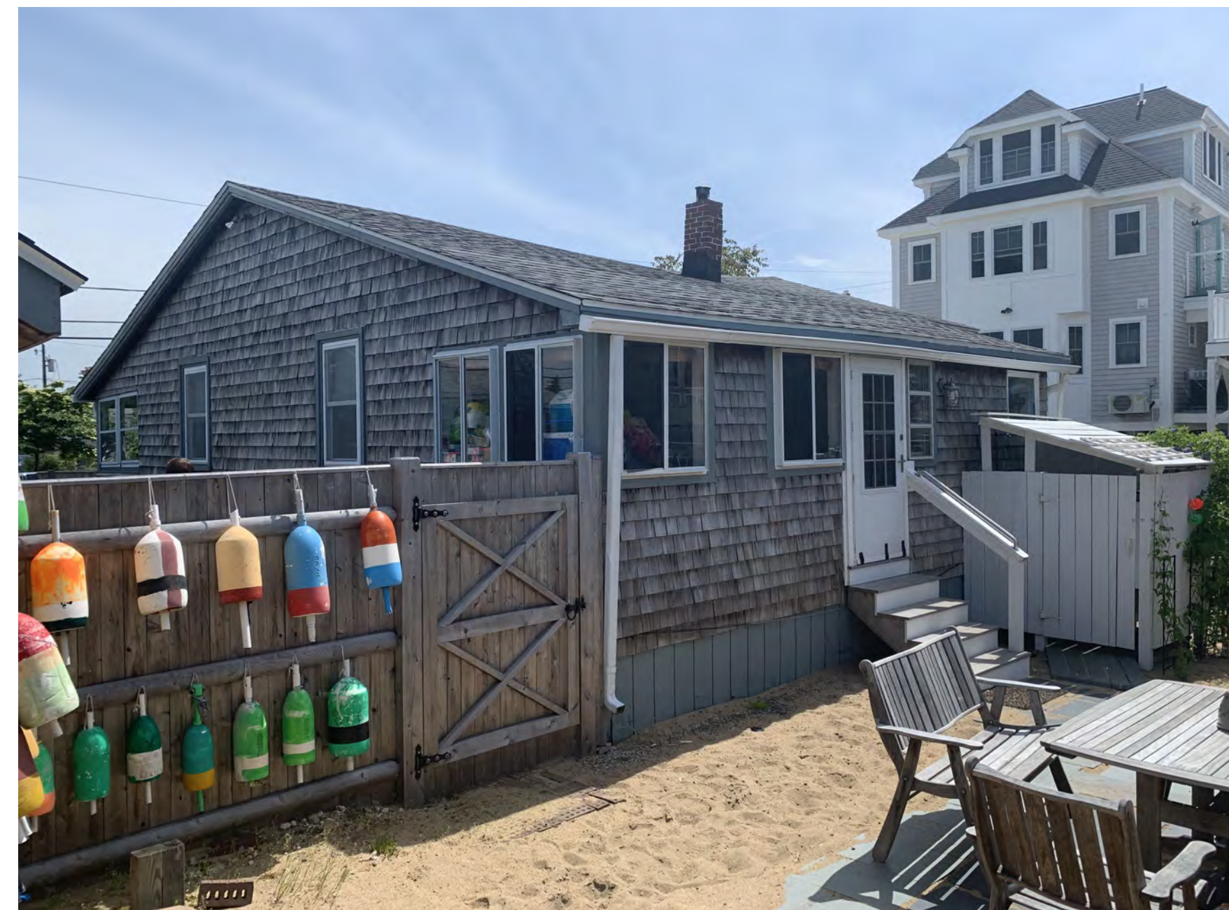
Note sand area in back with stone patio to be removed
