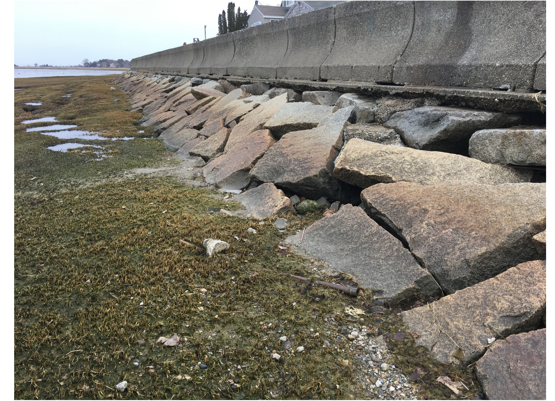
View along seawall
