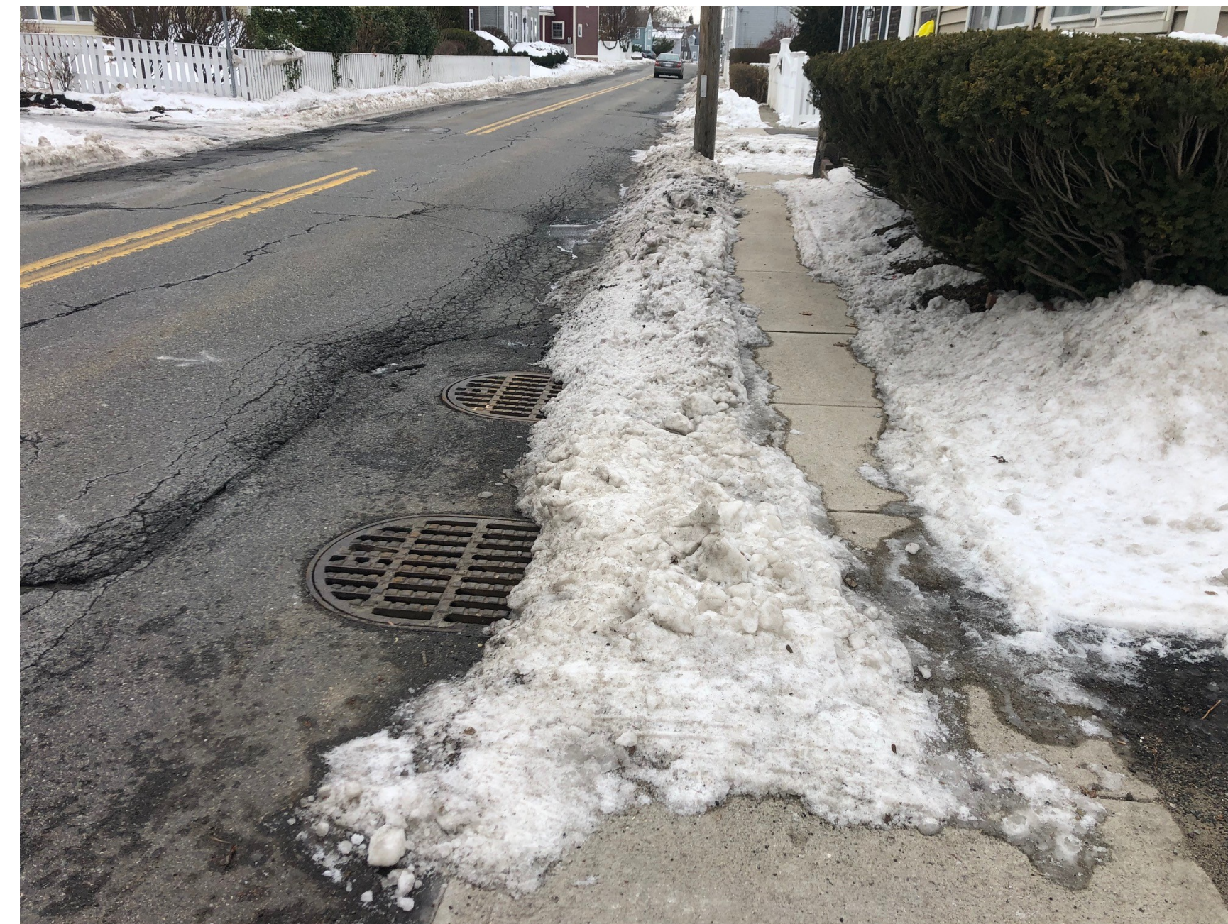
View along water street. Note storm drains. Line to be replaced
