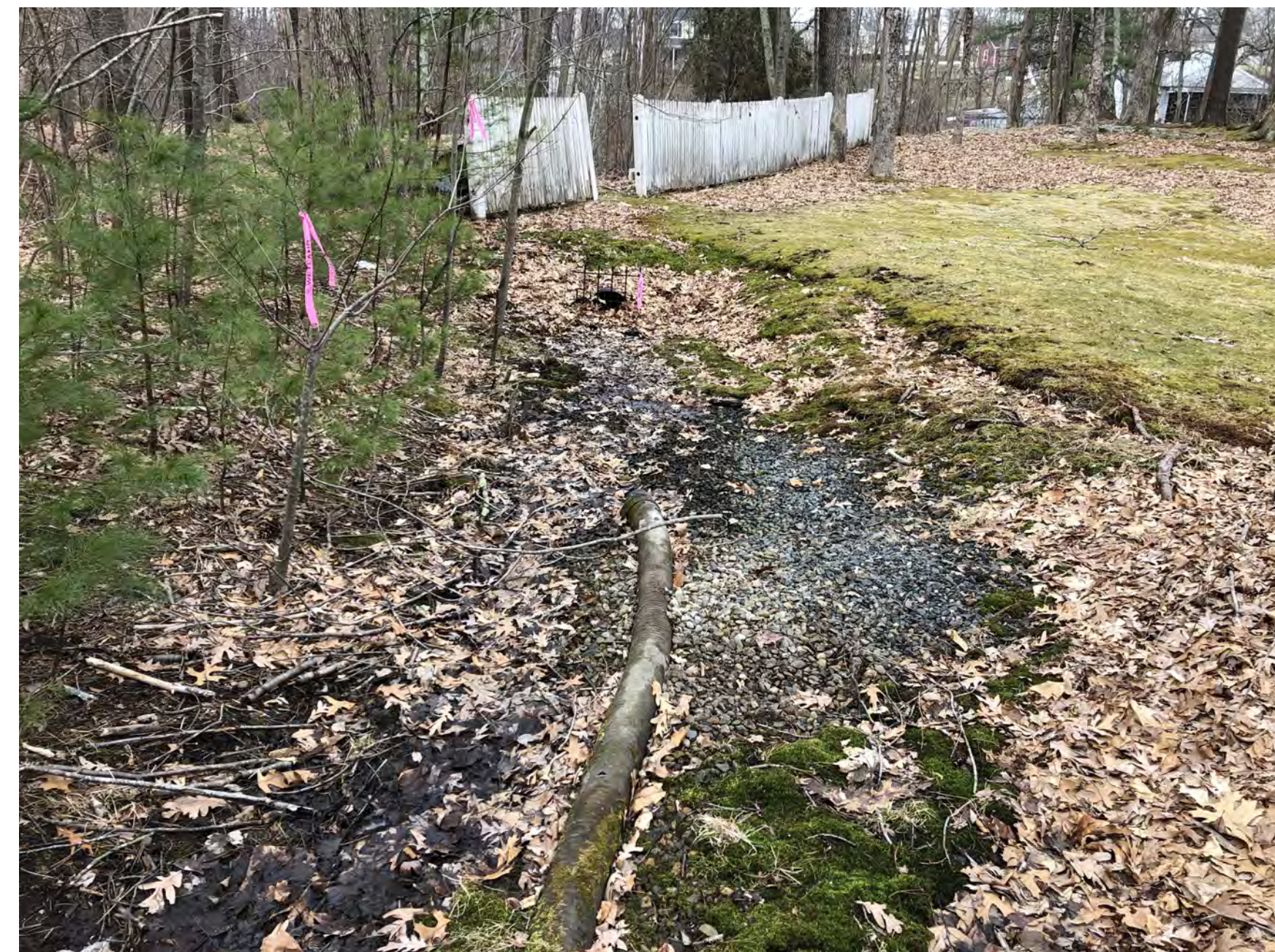
Wetland area drains into pipe
