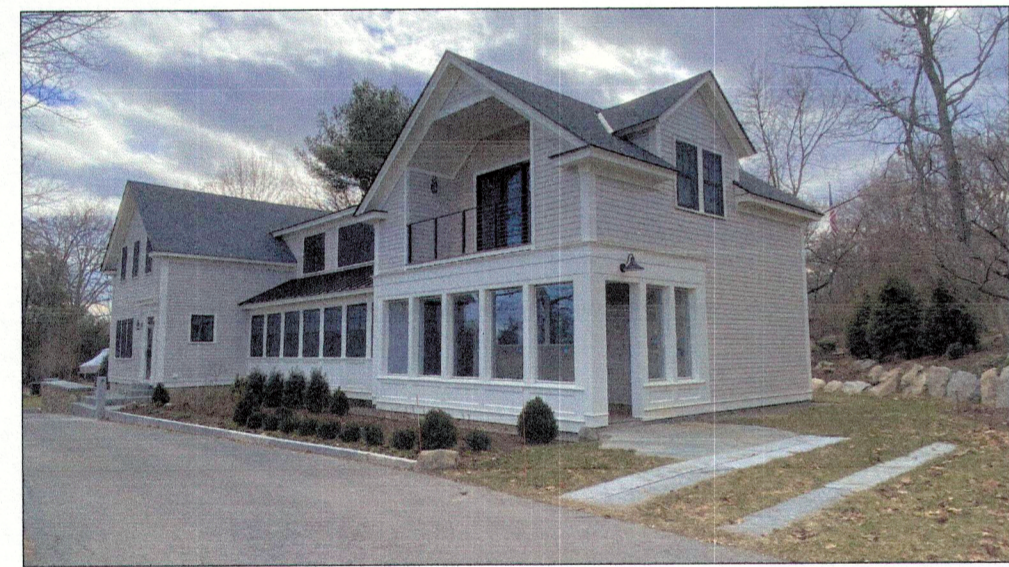
NORTHERLY BUILDING VIEW FROM JEFFERSON CT
