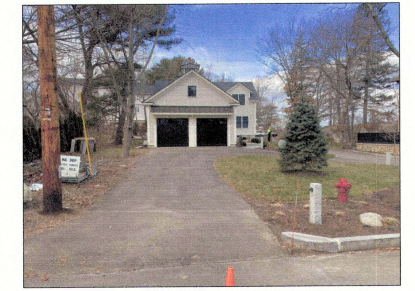
SOUTHERLY BUILDING VIEW FROM JEFFERSON ST
