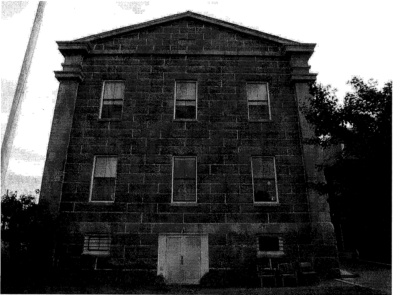
(iii) 7/27/2013 View of north façade, Gregory Colling
