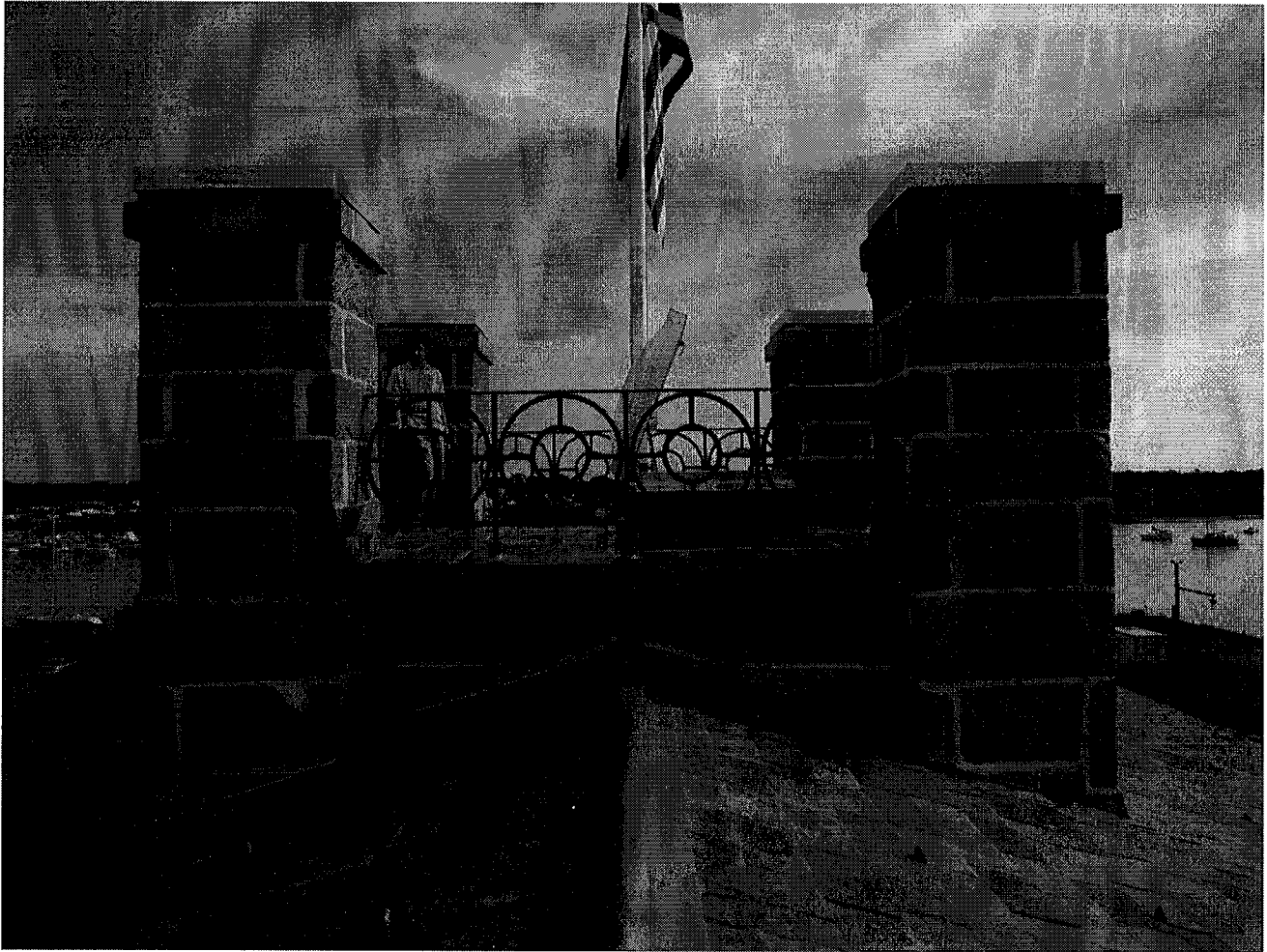
(vi) 7/24/2013 Observatory guardrail detail, Gregory Colling
