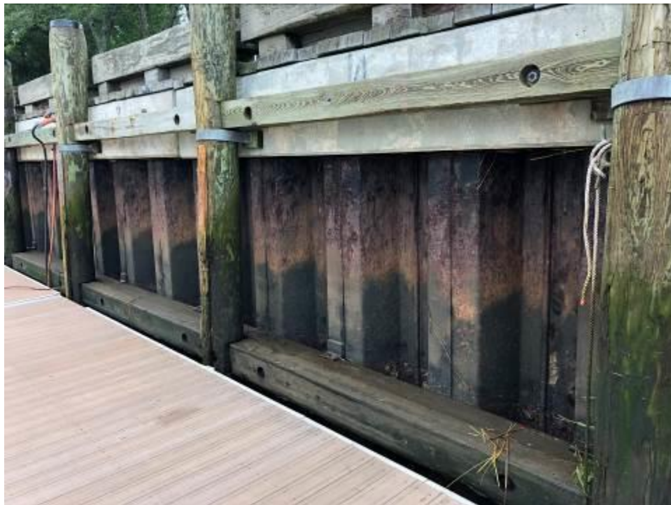
Existing Center Embayment – Typical conditions
