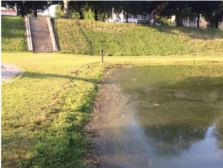
Lack of an edge is compromising surrounding walkways. Water should be kept at a constant level with well and outlet.
