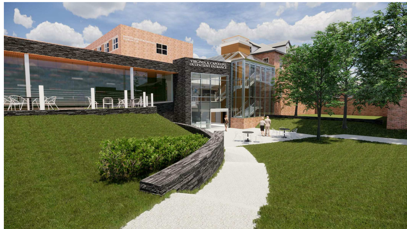
VIEW OF OUTPATIENT ENTRANCE FROM DROP-OFF
