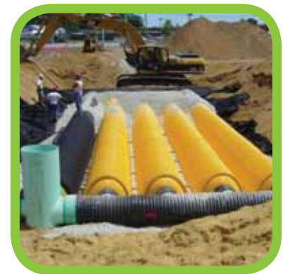
StormTech Isolator Row with Overflow Spillway (not to scale)
