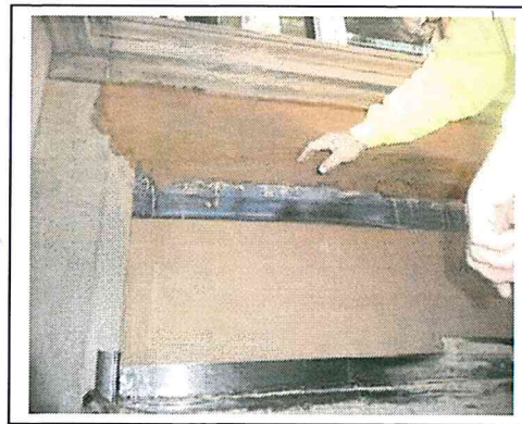
Starting to install the repair
