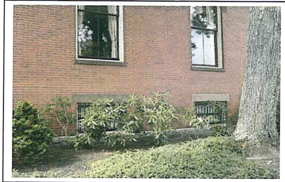
Basement lintels use salvaged stone
